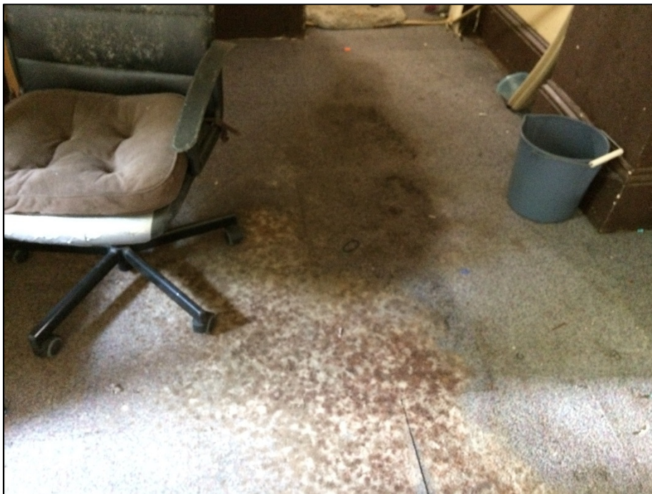
Photo 2: Signs of water damage on the first floor of the building.
