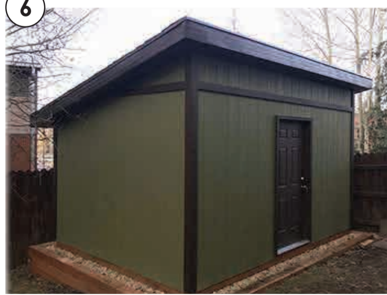
6 10' X 10' SECURED SHED
