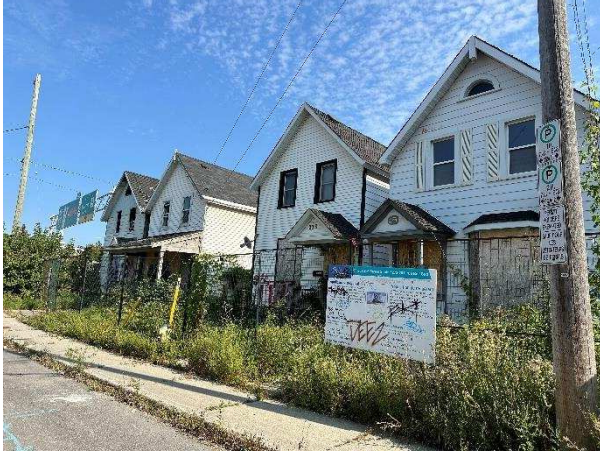
Photo 1: 269, 271, 273 and 275 Bell St S.
