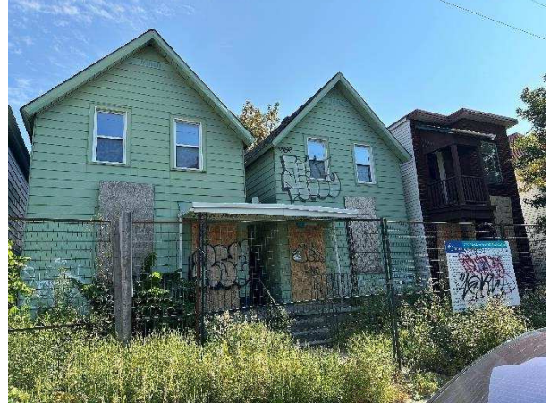
Photo 2: 277, 279 and 281 Bell St S
