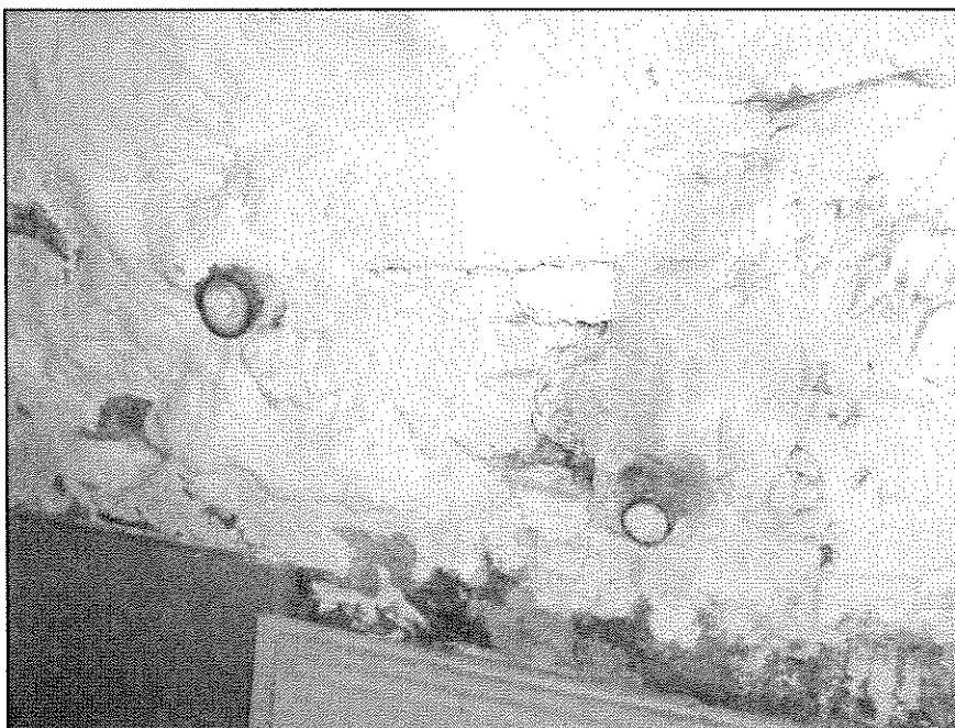
Photo 8 - Vent fill pipes in the basement wall of 136 Bank Street.
