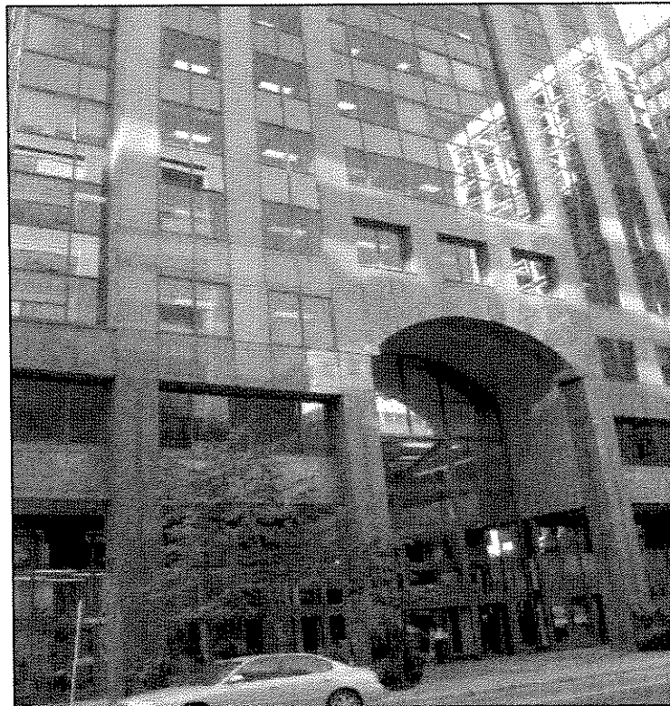
Photo 2 - 333 Laurier Avenue office tower, from Laurier Avenue.
