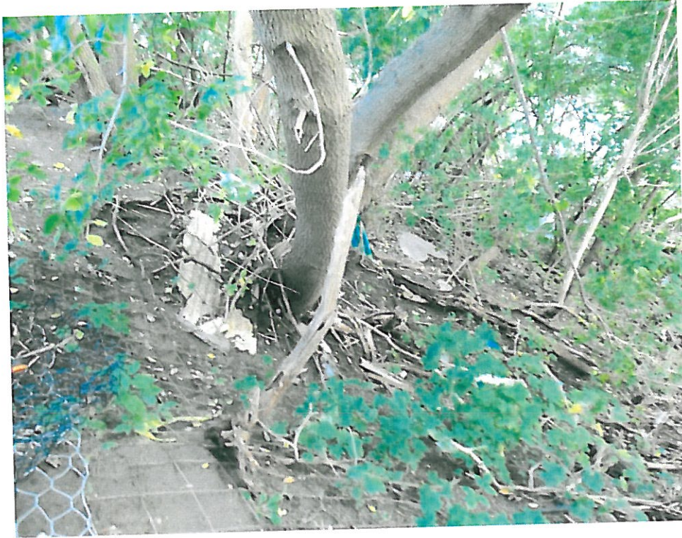
Photo 4. View of crest of slope looking north.
