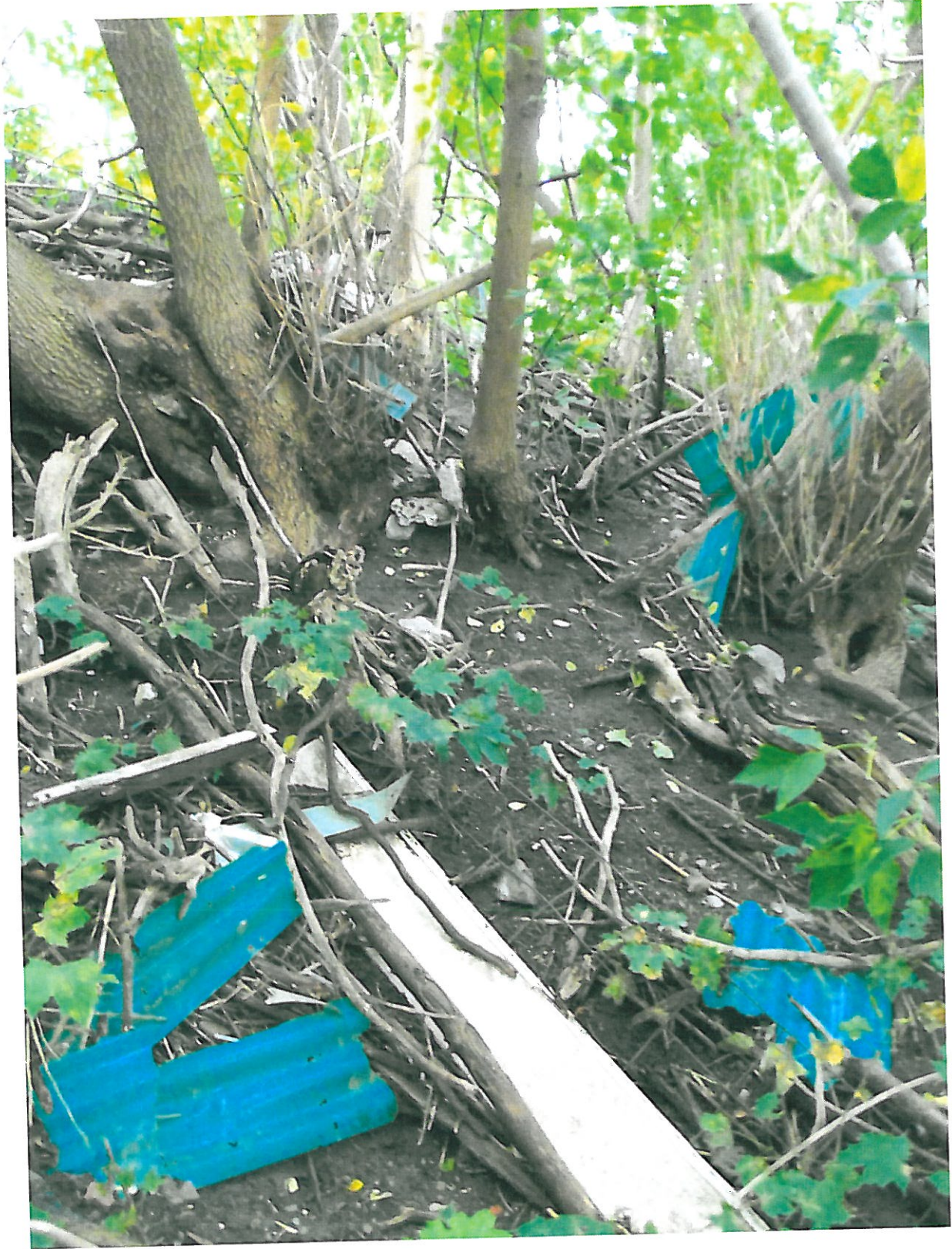
Photo 3. Close-up of slope near the crest
