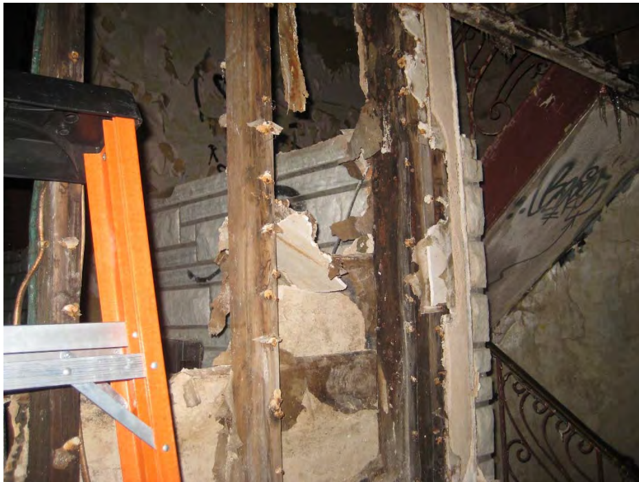
Photograph 14: View of the house.
