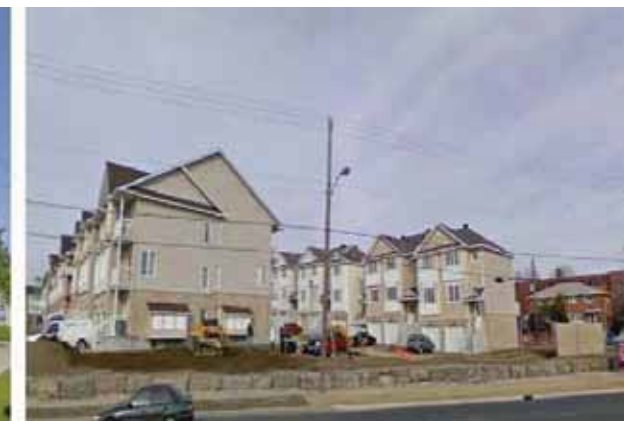
FIGURE 16: TOWNHOUSES AT MERIVALE AND CALDWELL
