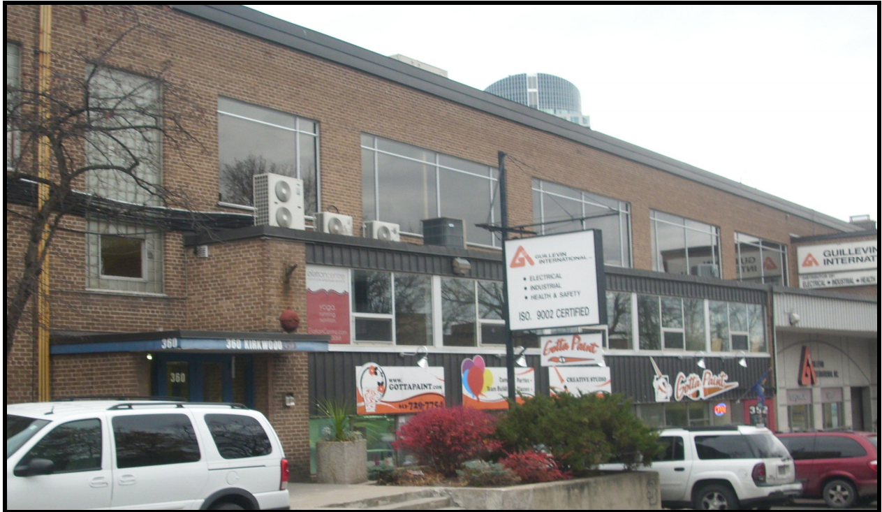
Photograph 3: East wall of southern portion of the building, facing northwest.
