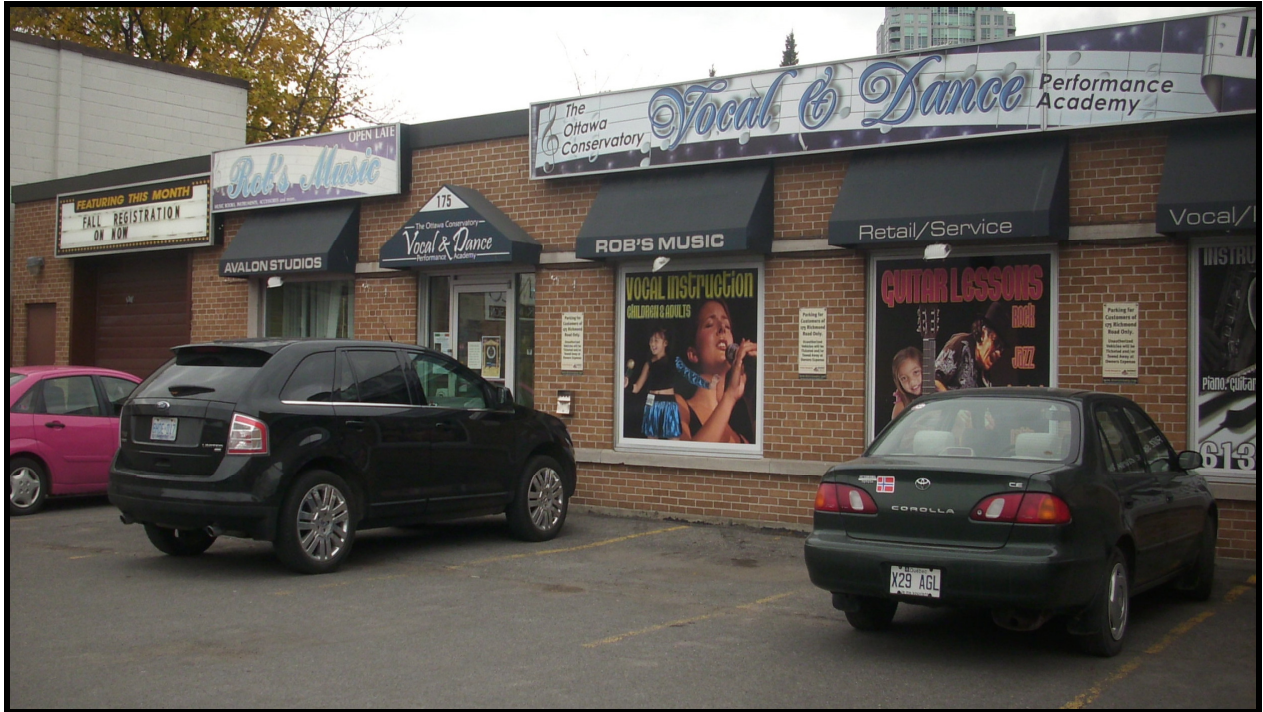
Photograph 1: South wall of western portion of the building, facing north.
