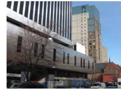
North side of Gloucester looking east towards Metcalfe
