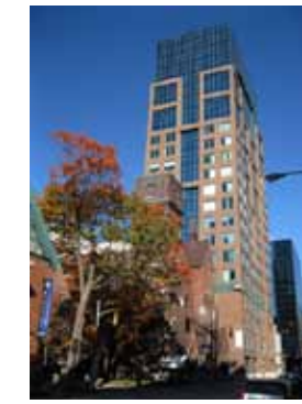
Looking toward the northwest corner of Metcalfe and Gloucester
