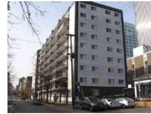
Looking west along Nepean from the front of the site
