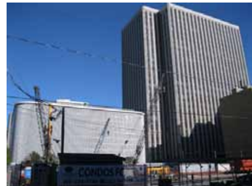
Looking toward the northeast corner of Metcalfe and Nepean, with future Tribeca development in foreground
