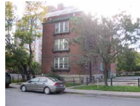
Looking south across Nepean at the adjacent building to the east
