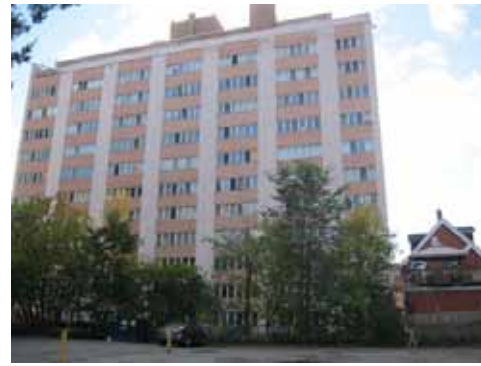
Looking southeast from the site
