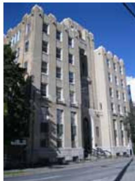
Looking toward the southwest corner of Metcalfe and Nepean
