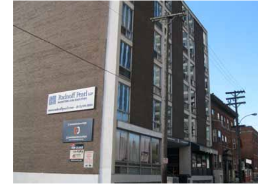
South side of Gloucester looking west, between Metcalfe and O'Connor
