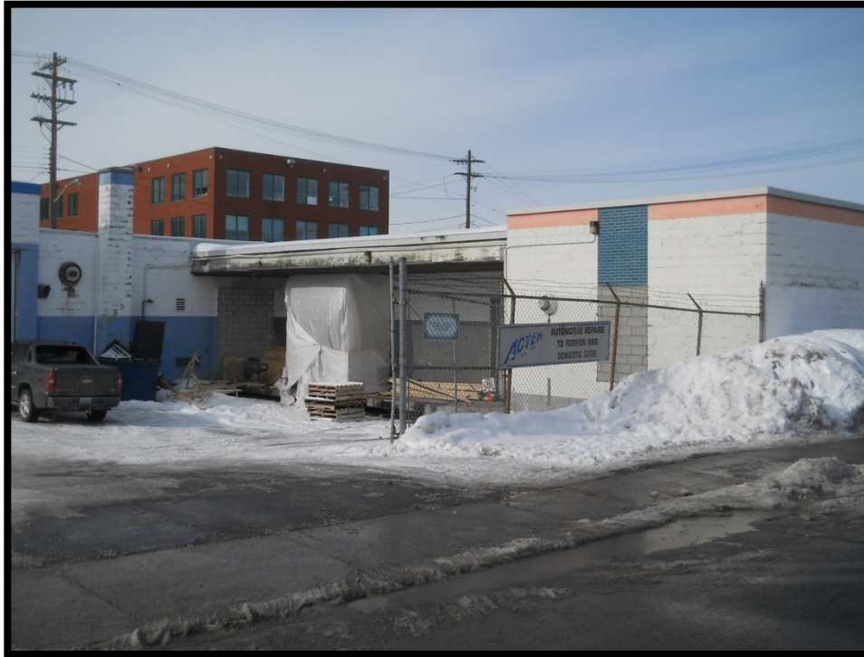
Photograph 3: View of loading area to the south of the commercial portion of the building. View is looking northwest.
