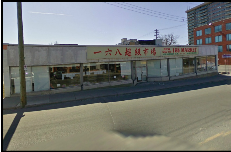
Photograph 1: (Google Street View) View of the north side of the site looking south. Photograph illustrates the vacant commercial (north) portion of the subject building.
