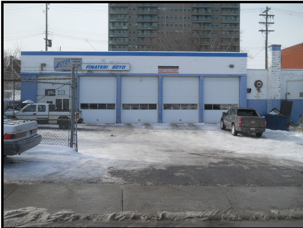
Photograph 2: View of the automotive service garage (south) portion of the subject building, looking west. Photograph illustrates the service bays of the automotive garage.
