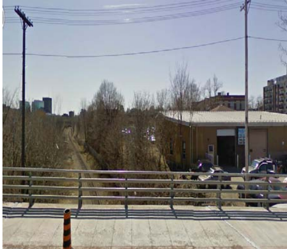
Somerset Street bridge and train tracks below.
