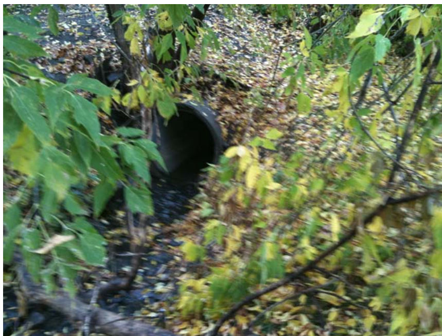
Photograph No. 4 Adjacent storm water culvert
