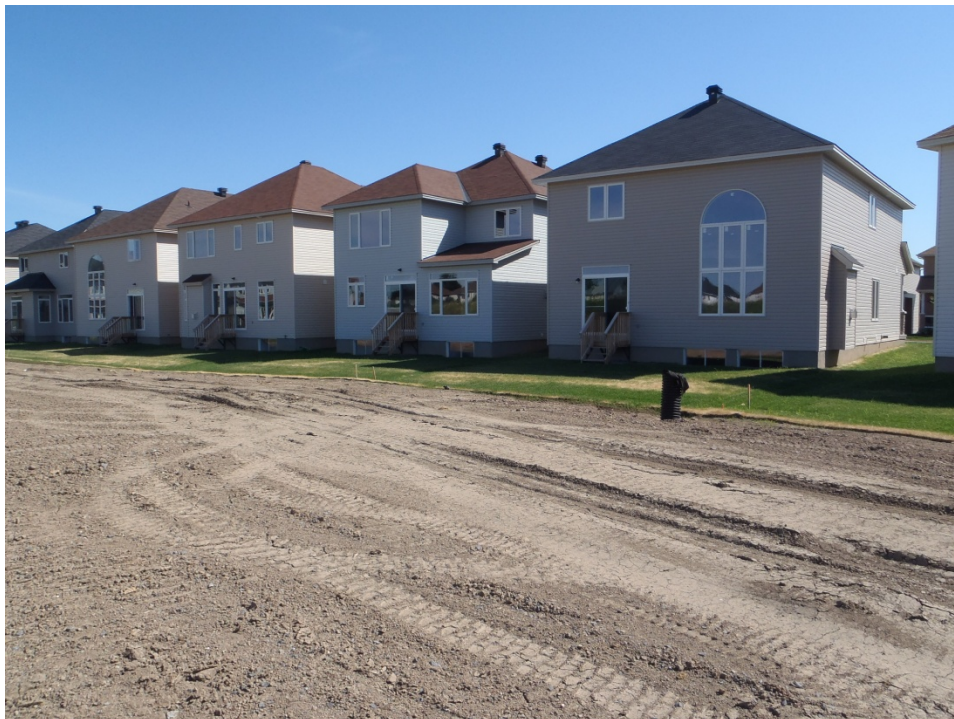
Photograph 2: Looking east towards townhouses on the east side of the Site.
