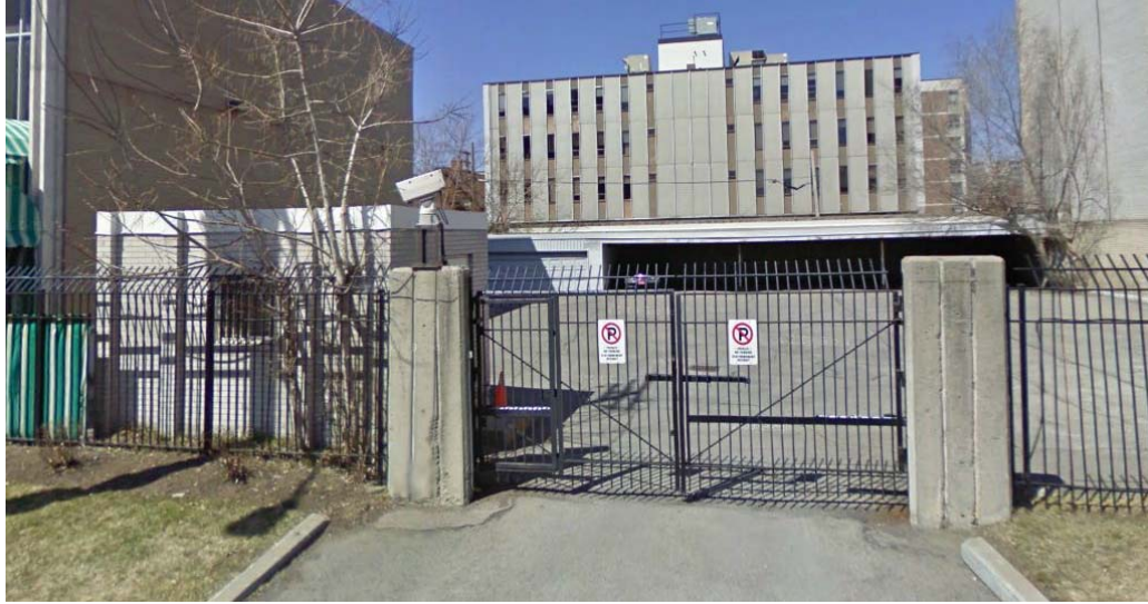
Figure 9: The guardhouse, fence, parking lot and garage on the eastern portion of the property at 215 McLeod Street, 2009. (Google Street View)
