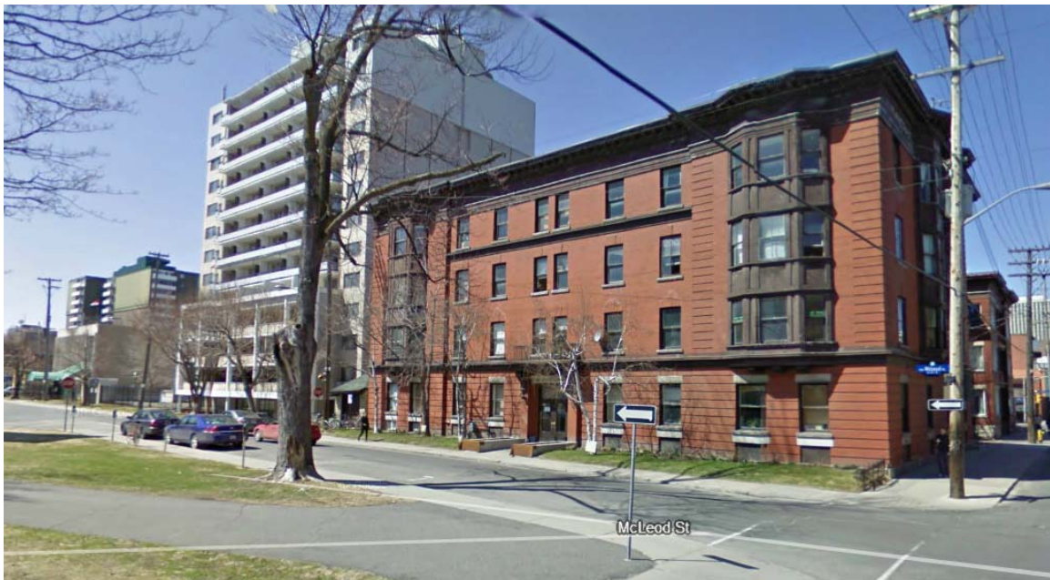
Figure 6: 191 McLeod Street at the corner of Elgin Street. The Embassy of Iraq is at the far left side of the image. The 13-storey 1960s apartment tower is located between the corner building and the Embassy, 2009. (Google Street View)
