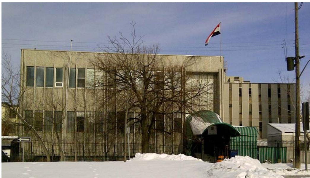
Figure 4: The front elevation of the office building for the Embassy of Iraq on the western portion of the property at 215 McLeod Street. (Contentworks, 29 February 2012)
