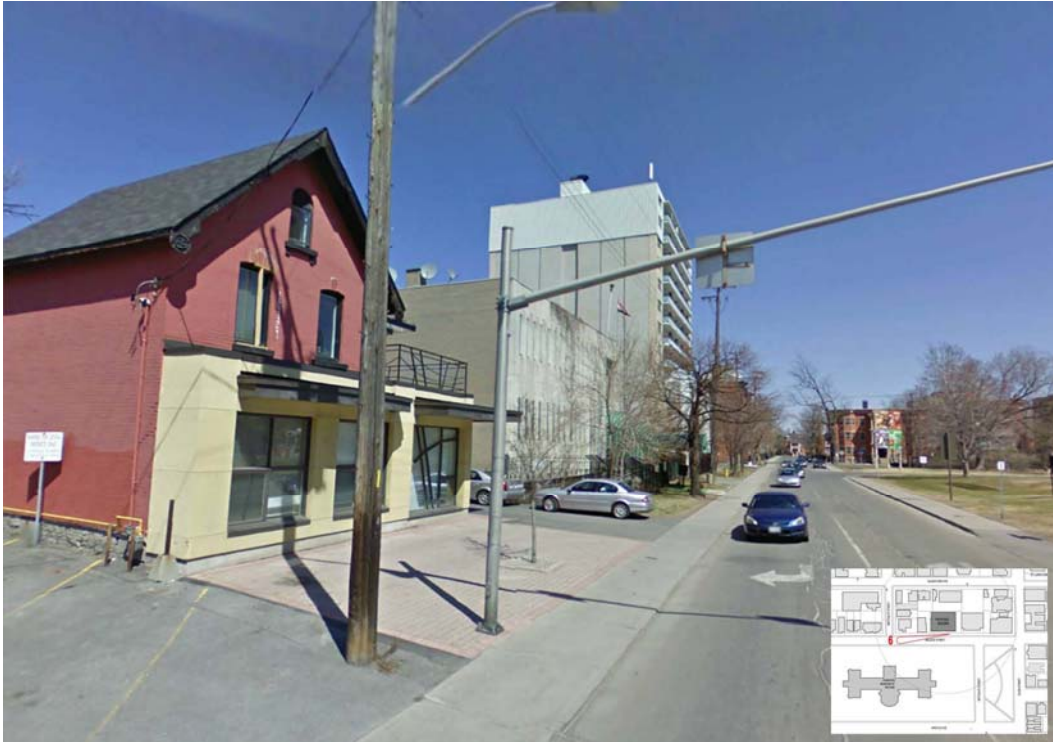
Figure 7: 223 McLeod Street (left) and the Embassy of Iraq (centre). (Julian Jacobs Architects, 20 December 2011.)
