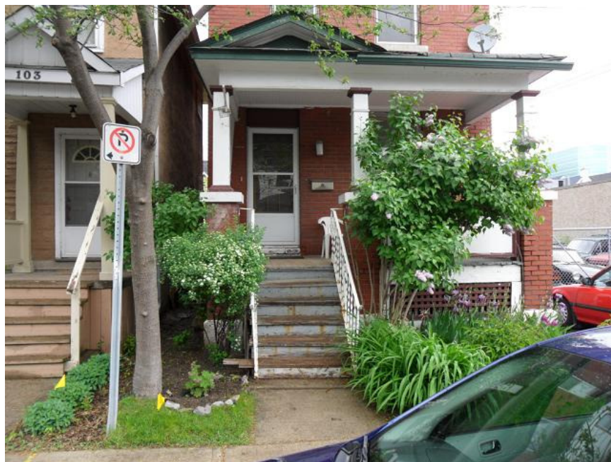
Photograph 2: Residential dwellings at 99 and 103 Norman Street, facing north.
