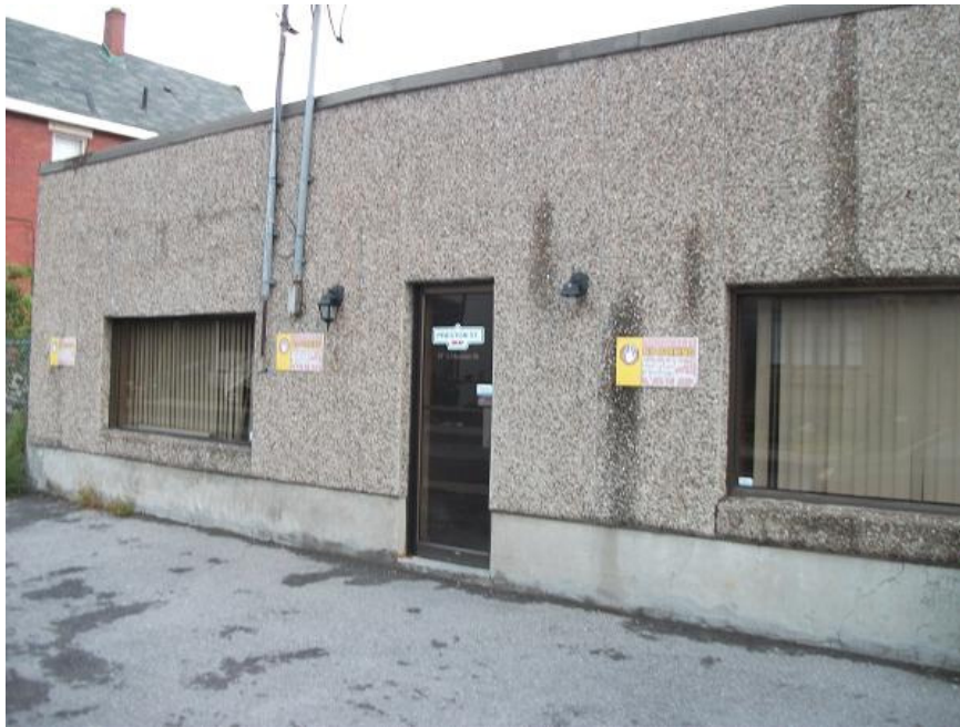
Photograph 4: Office building at 97 Norman Street, facing northwest.
