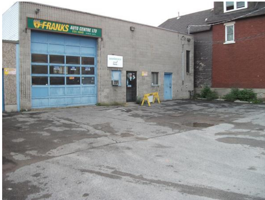
Photograph 5: Former garage at 95 Norman Street, facing northeast.
