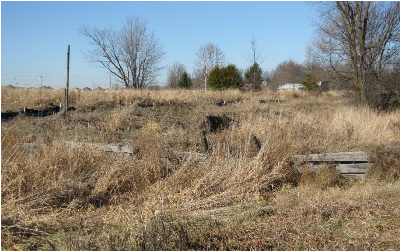
Plate 3: Small bridge built with left over materials, crossing between sections 6G and 6D, looking north from the boundary of 6G and 6D.
