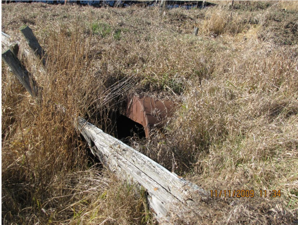
Plate 14: An old boiler or oil tank being re-used as a culvert in the bridge between sections 6D and 6G, looking northwest.
