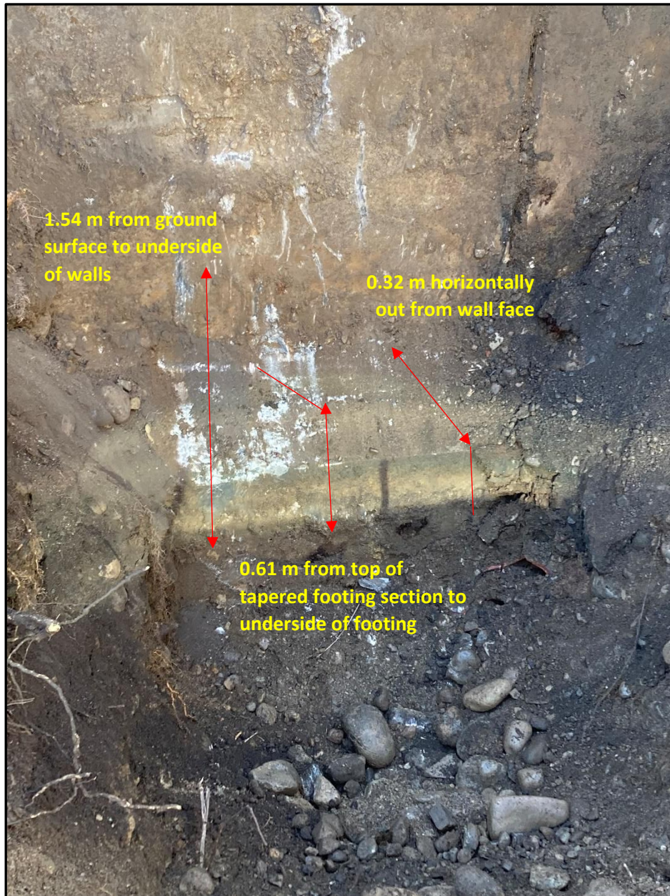
Photo 5 – Details of TP2-22, of the existing retaining wall abutment system for adjacent section of Somerset Street from field program dated April 2022. Wall abutment placed over engineered granular fill.
