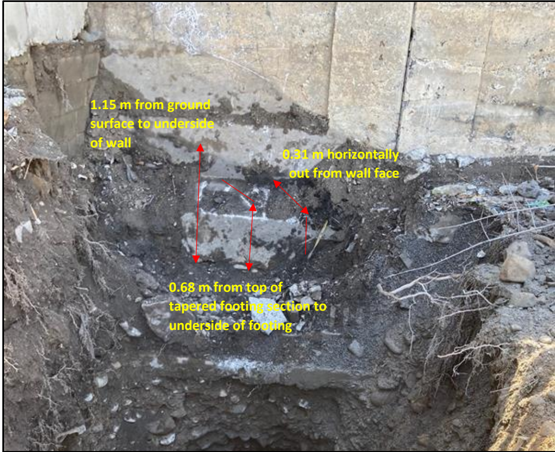
Photo 4 – Details of TP1-22, of the existing retaining wall abutment system for adjacent section of Somerset Street from field program dated April 2022. Wall abutment placed over engineered granular fill.
