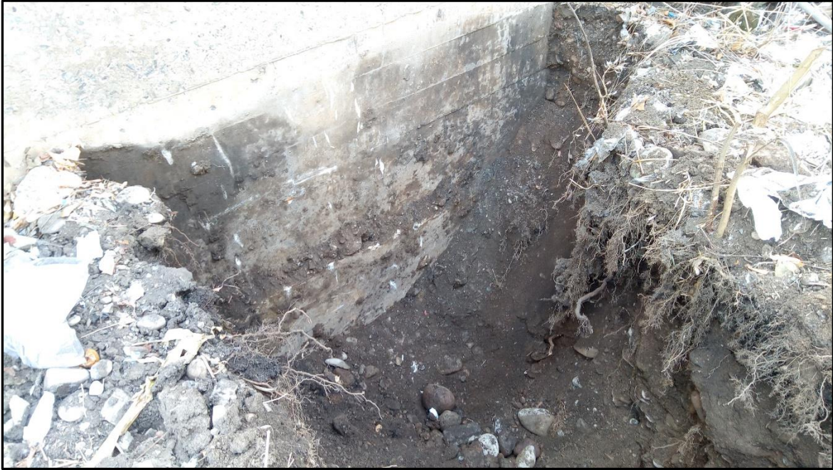
Photo 1 – Test pit at adjacent retaining wall along Somerset Street.
