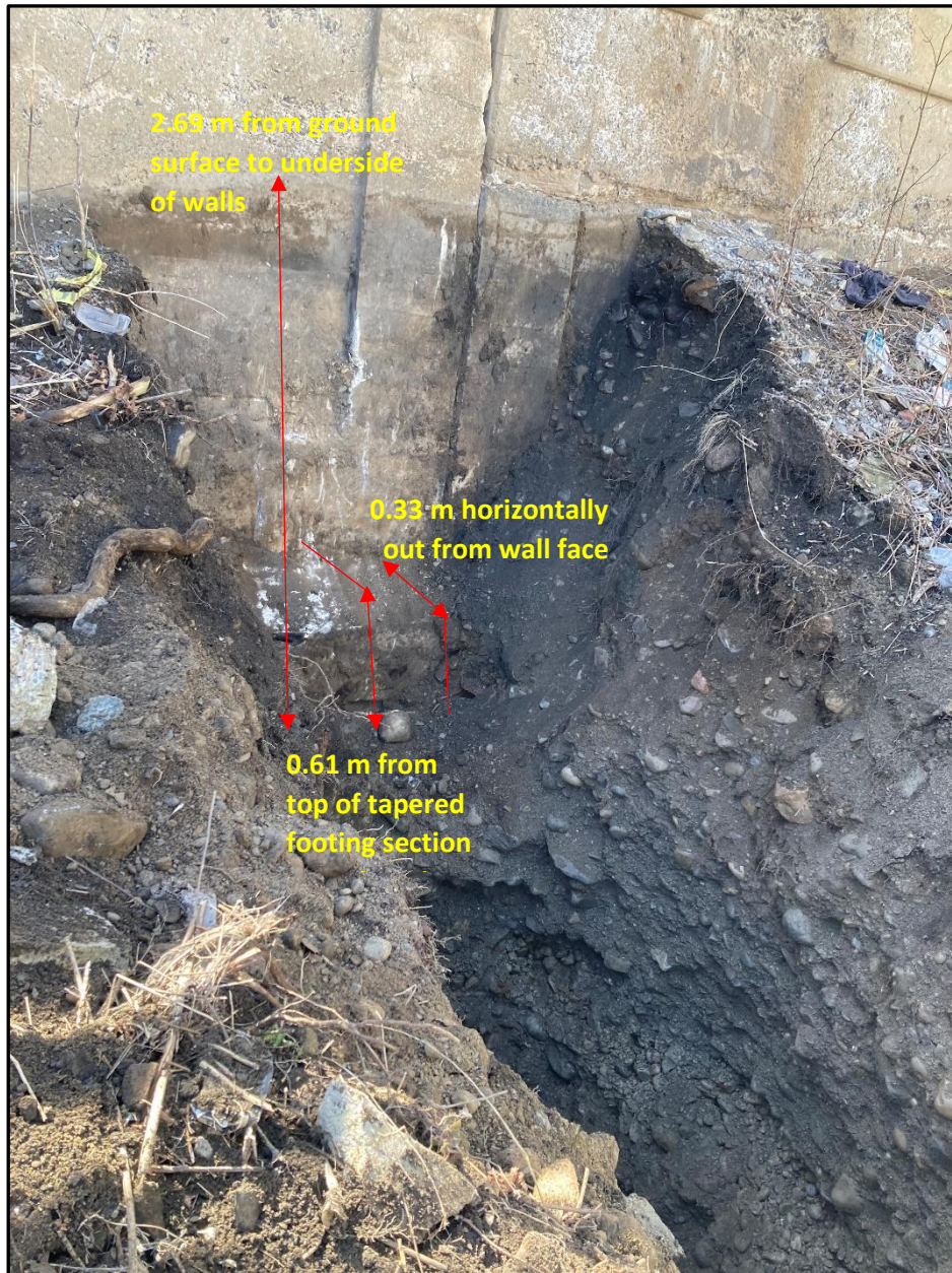
Photo 6 – Details of TP3-22, of the existing retaining wall abutment system for adjacent section of Somerset Street from field program dated April 2022. Wall abutment placed over engineered granular fill.
