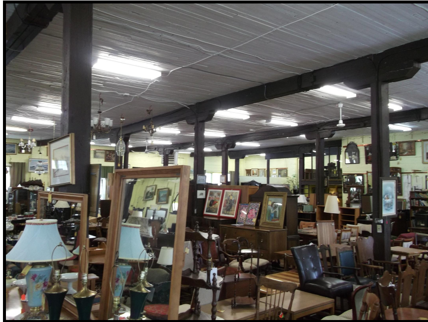
Photograph 1: Interior of second storey of subject building (A Fine Thing Antiques).
