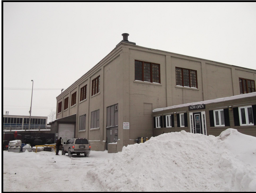
Photograph 5: Subject building, facing southwest from Spruce Street.
