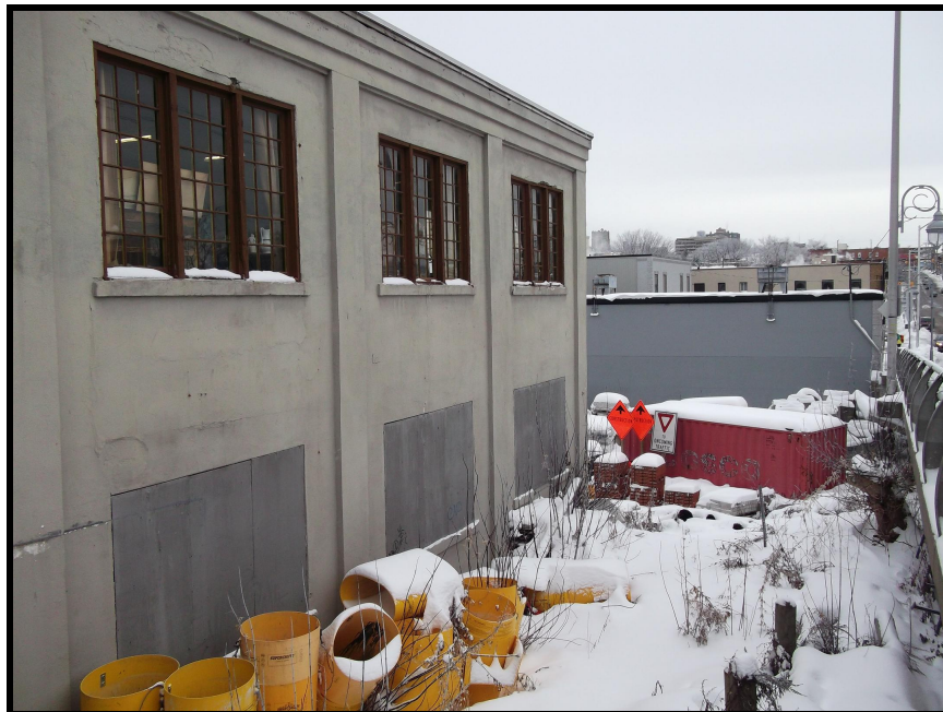
Photograph 2: Facing north from Somerset Street West along east boundary of subject building, showing Domicile construction materials storage.
