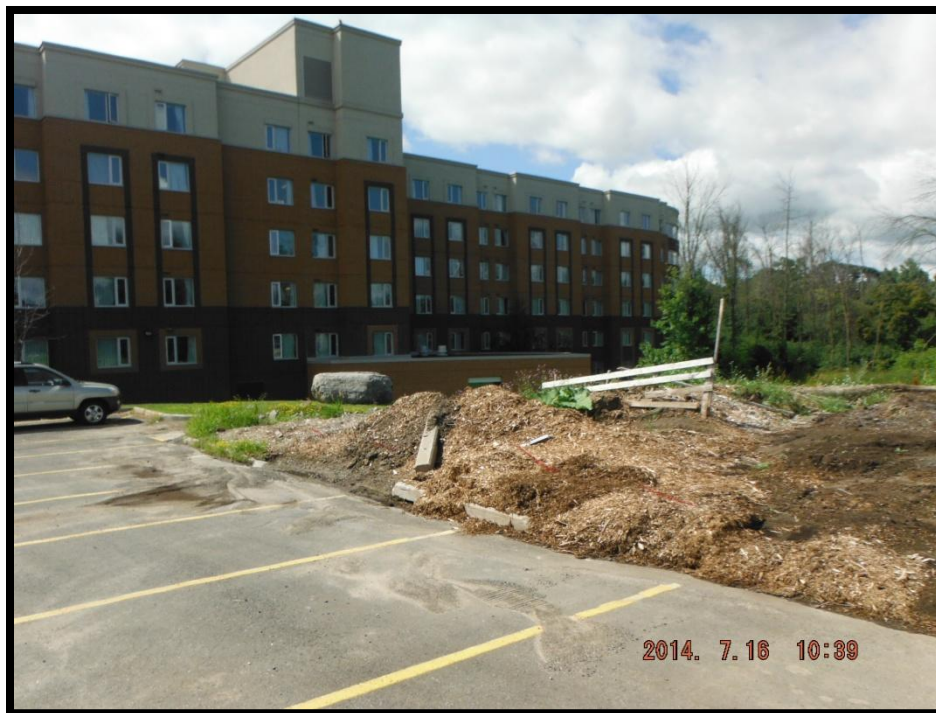
Photograph 2: View of southwest portion of the parking lot. Photograph depicts fill at apex of the escarpment, as well as, the location where surface sheet flow is diverted.
