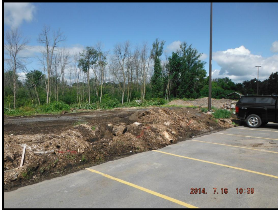
Photograph 3: View of top of escarpment on west side of parking area. Photograph illustrates fill on top of escarpment.
