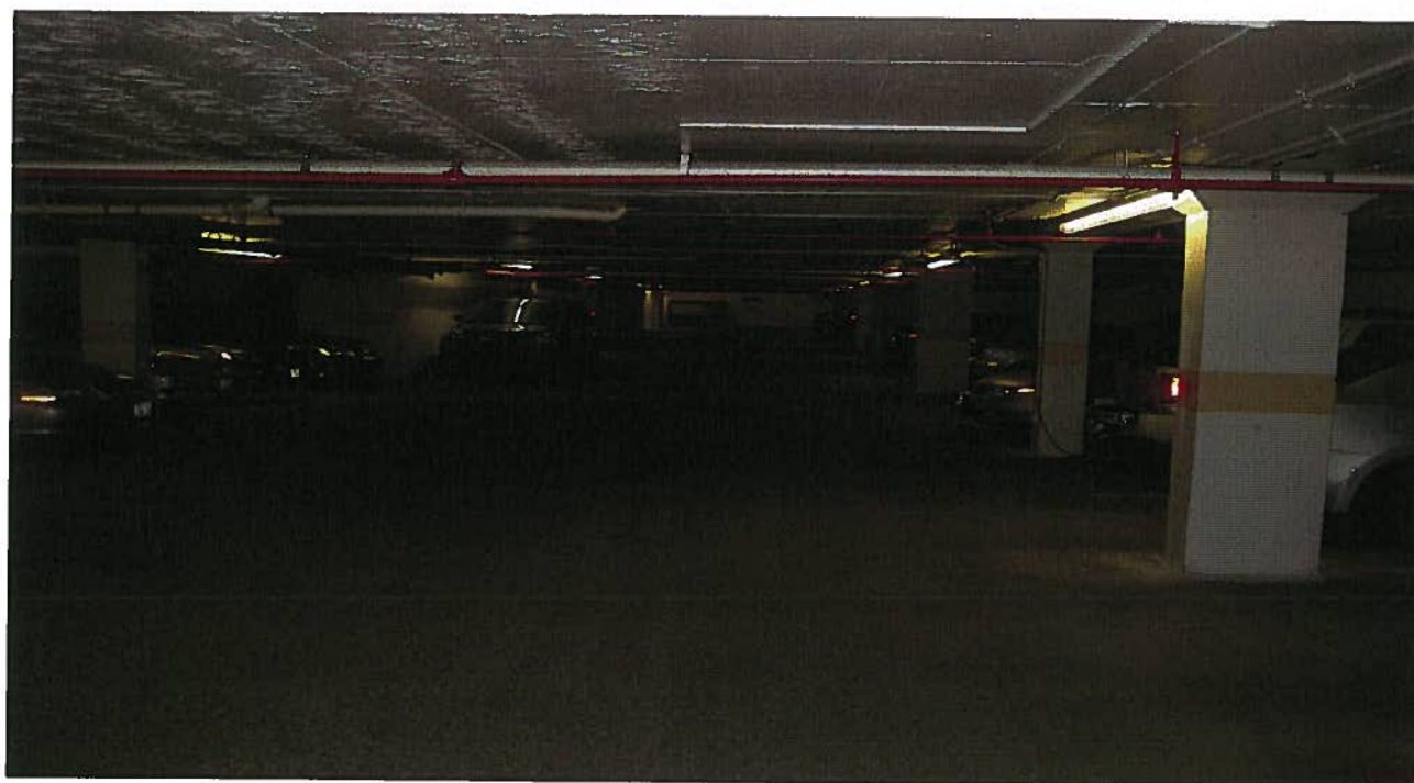
Photograph 14: Typical underground parking garage lane under 361 Queen Street.
