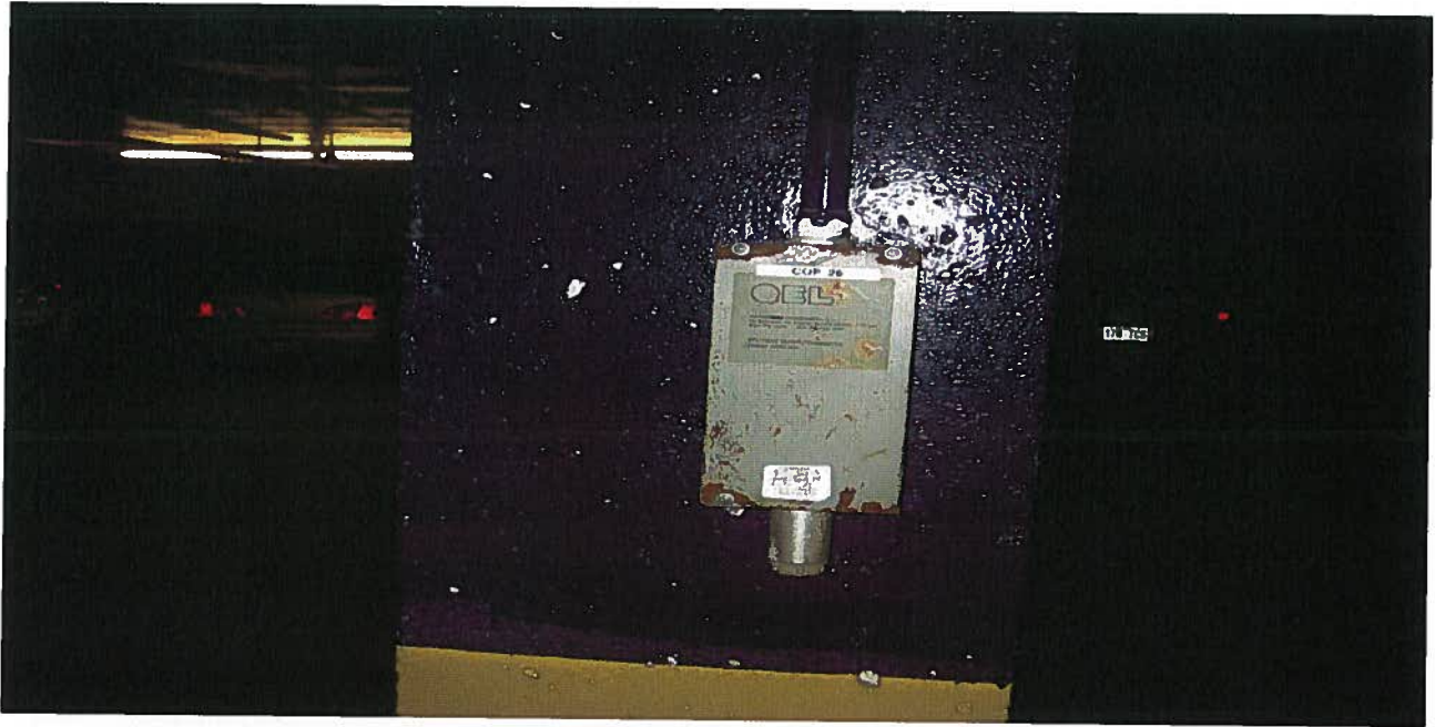
Photograph 11: One of several CO detectors observed on the underground parking lot columns.
