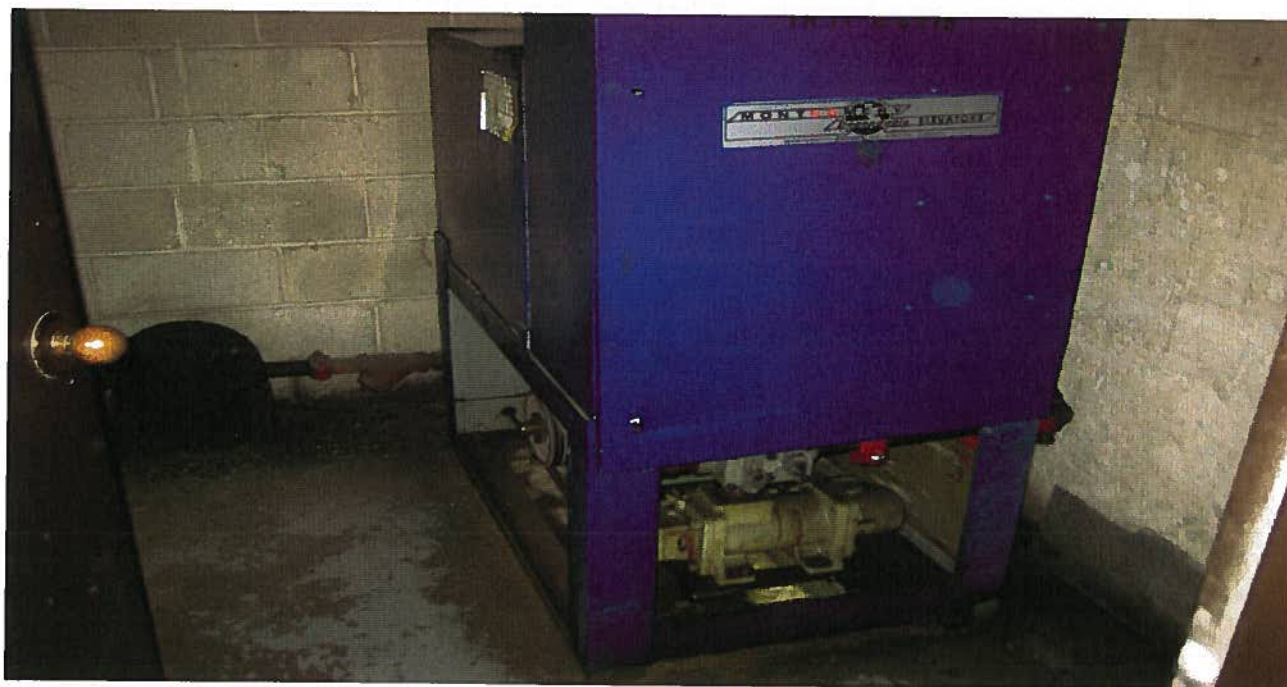
Photograph 10: One of two hydraulic elevator tanks. There were no indications of leakage from the hydraulic tank.
