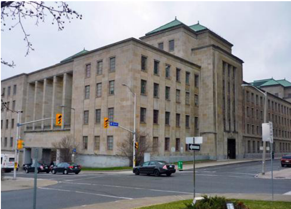
7. Corner view of West Memorial Building, 2011 (Source: Parks Canada Agency)
