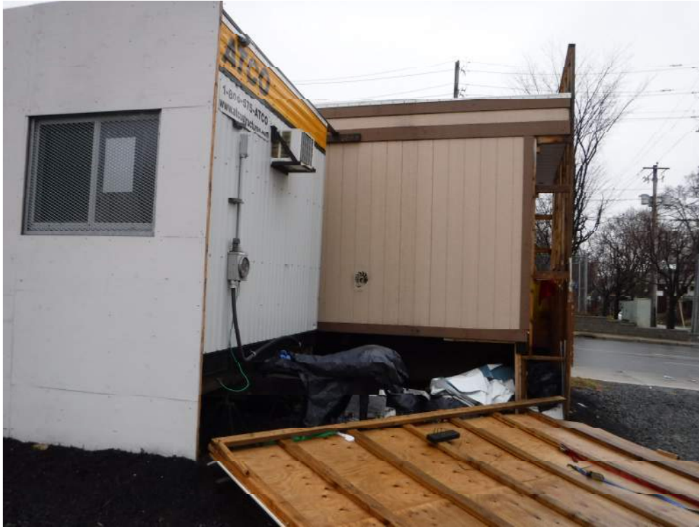
Photograph 3: Southwest corner of the on-site trailers.
