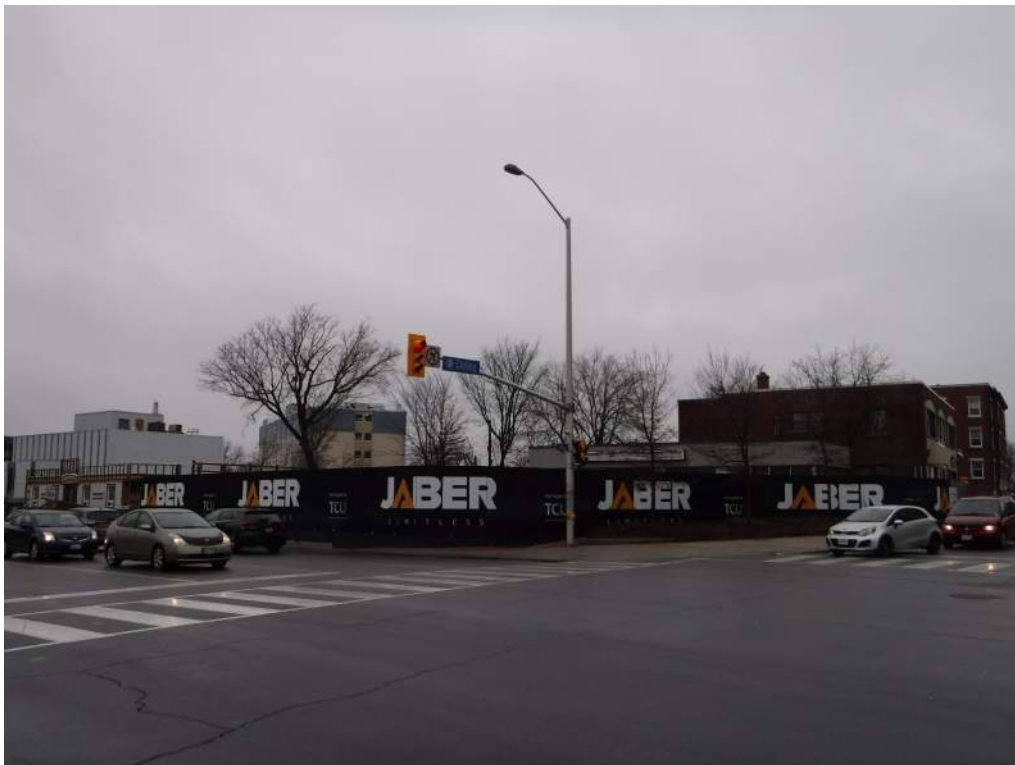
Photograph 10: Looking southwesterly across Bronson Ave. and Carling Ave. intersection at former auto repair/gas station located north of the Site.
