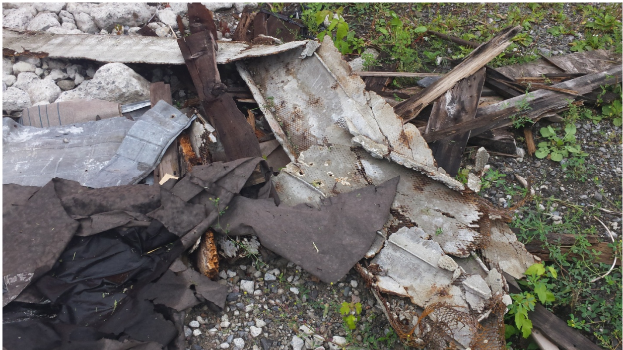
Photograph 4: Demolition debris including pieces of plaster lath and metal sheeting.
