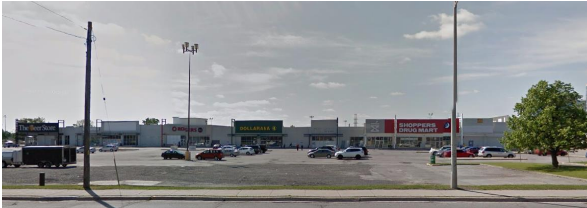
Exhibit 'B1' – Site Photo (Ogilvie Road frontage)
