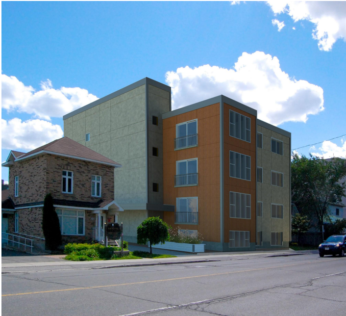
View of Site from North East
