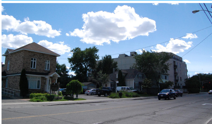
View of Site from North East
