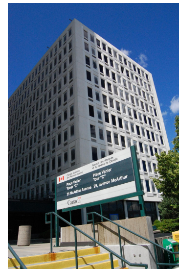
View of Adjacent Site, 25 McArthur Avenue
