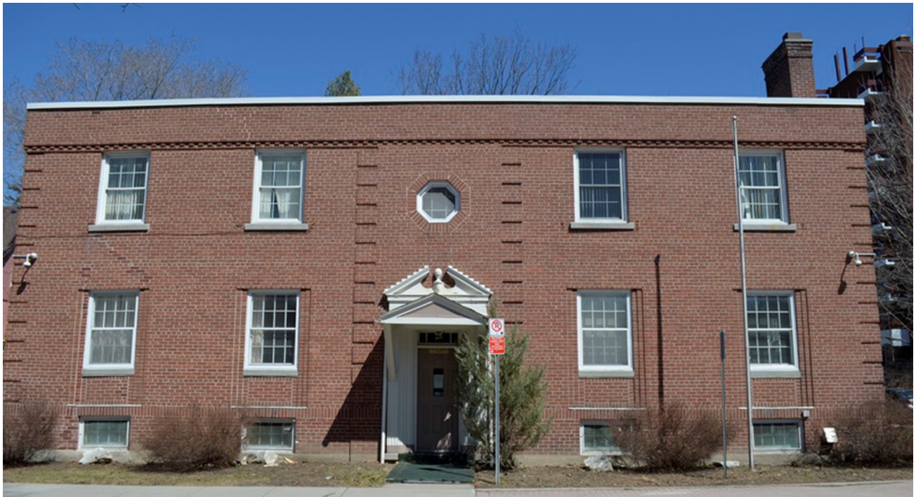
West (Main) Elevation at Cobourg Street.
