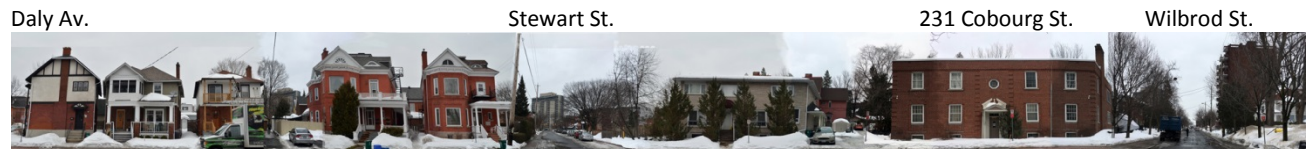
Streetscape – Cobourg Street East Side from Daly Avenue to Wilbrod Street.
