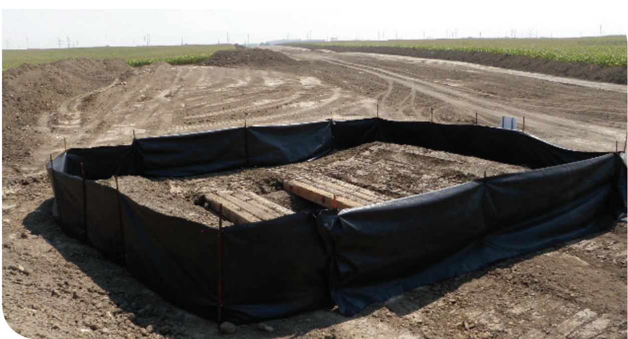
Cleaning station at construction site.
