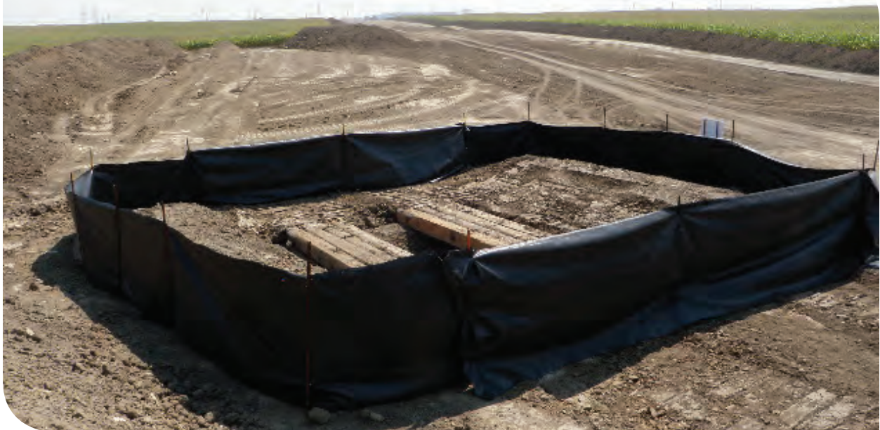
Cleaning station at construction site.
