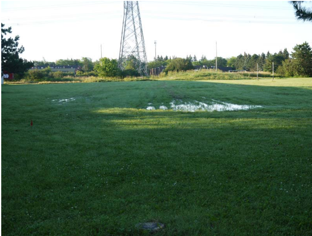
South facing view from site.
