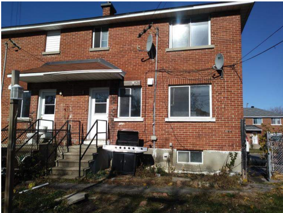
Photo 6: Rear exterior of 210 Prince Albert Street
