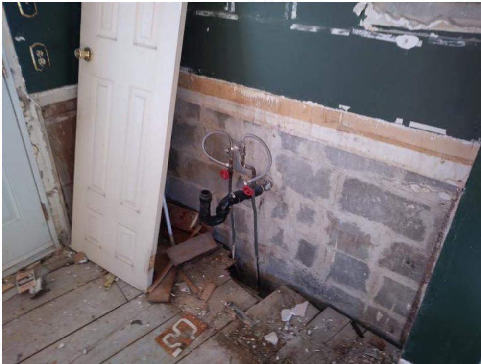
Photo 5: Plumbing fixtures in interior of 210 Prince Albert Street
