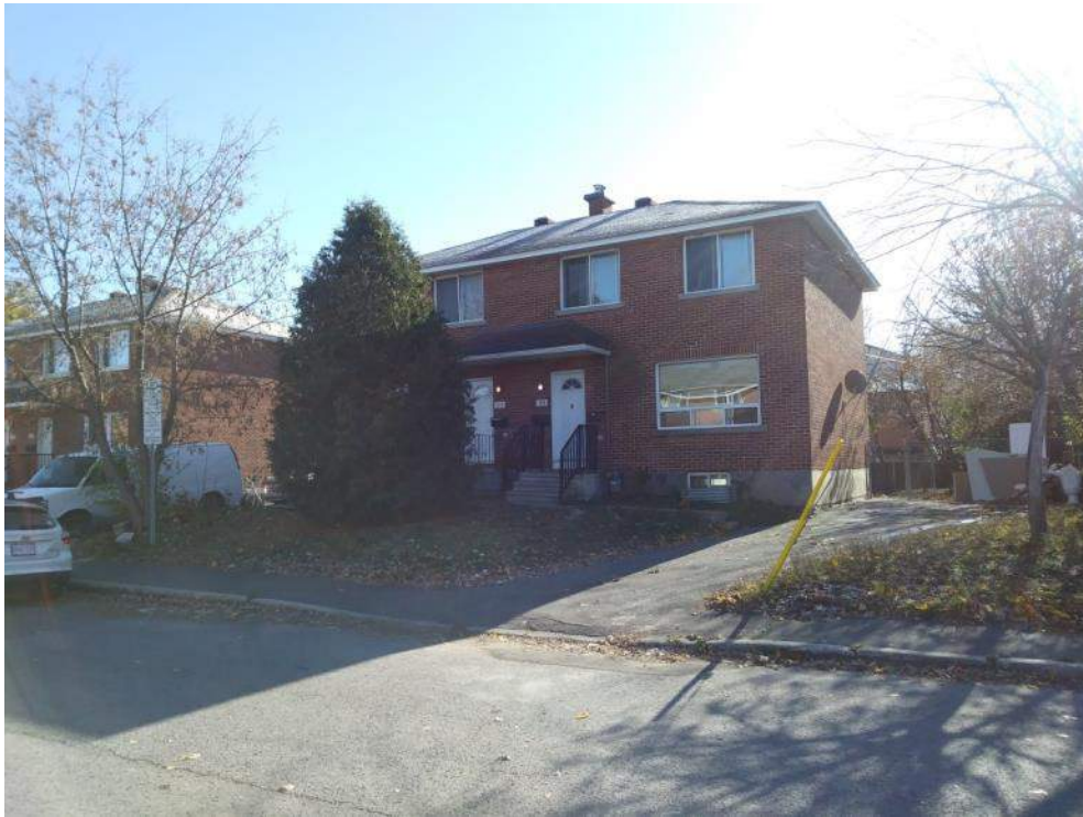
Photo 1: Exterior of Site
