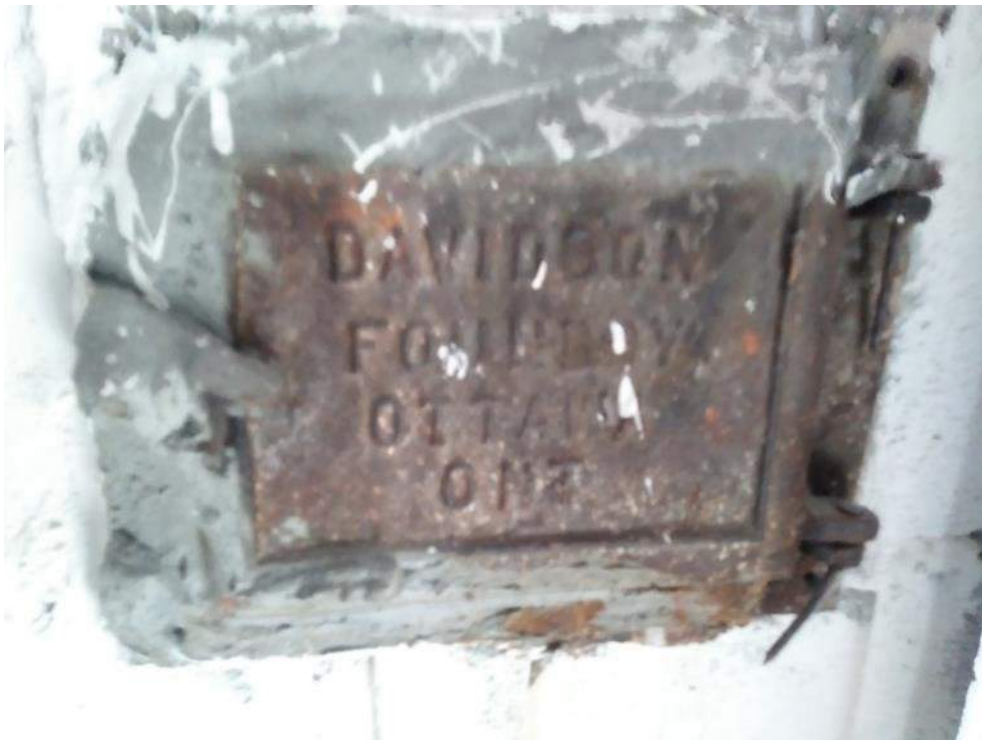
Photo 6: Ash cleanout port in 208 Prince Albert Street
