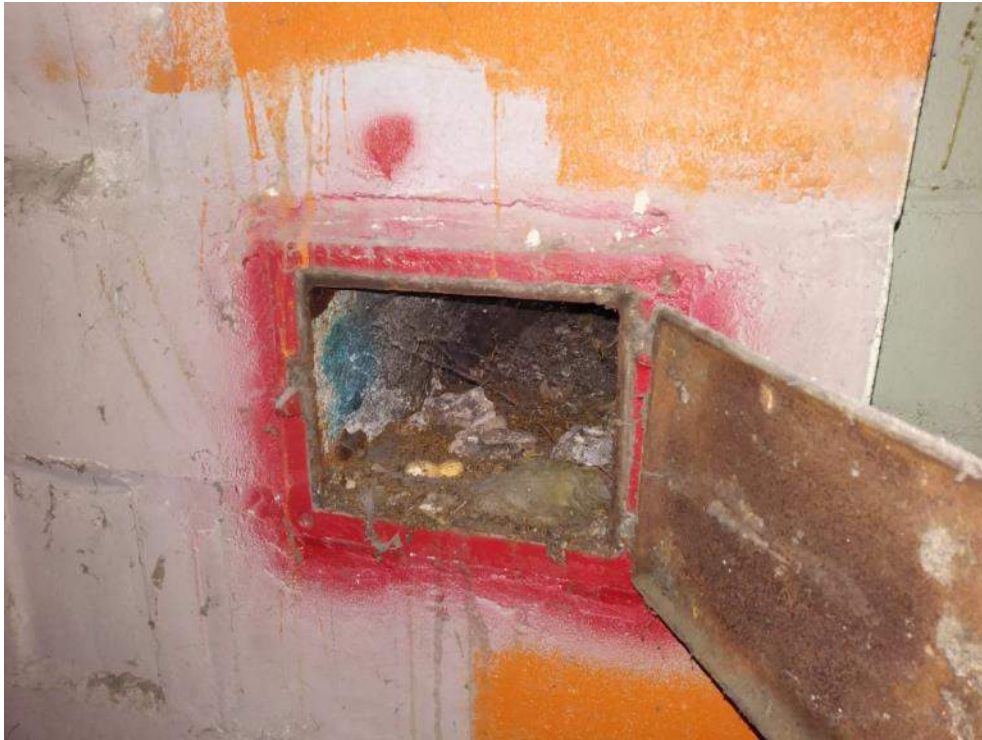
Photo 5: Ash cleanout port in 210 Prince Albert Street
