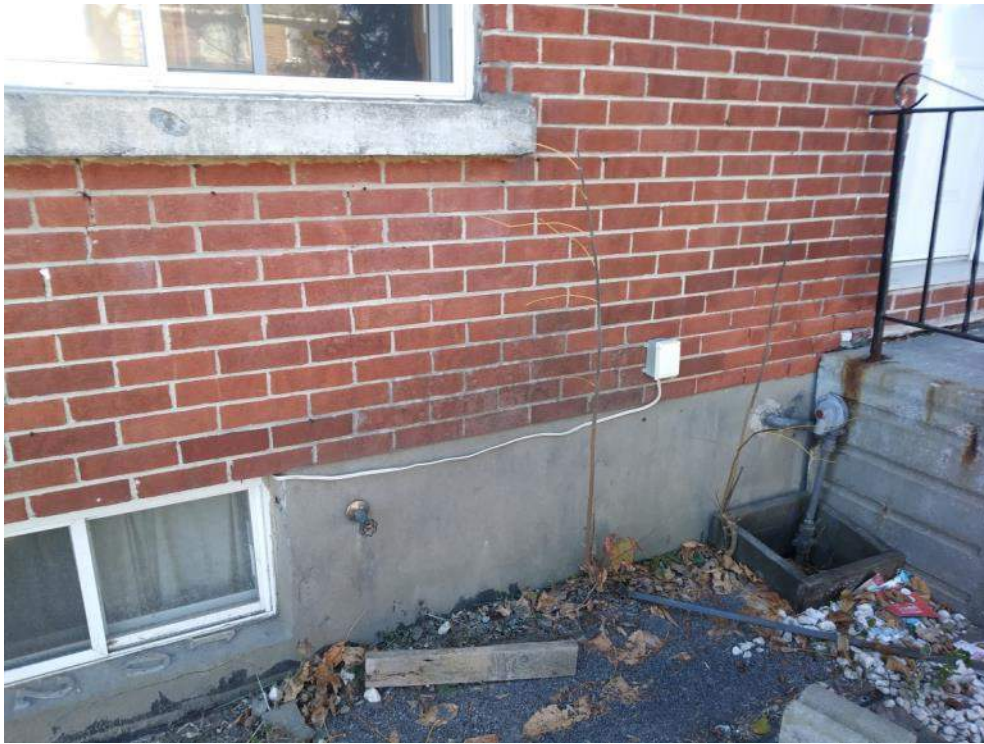
Photo 5: Rear exterior of 210 Prince Albert Street
