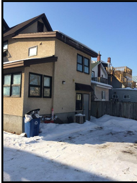
Photograph 3: View of the east building face.
