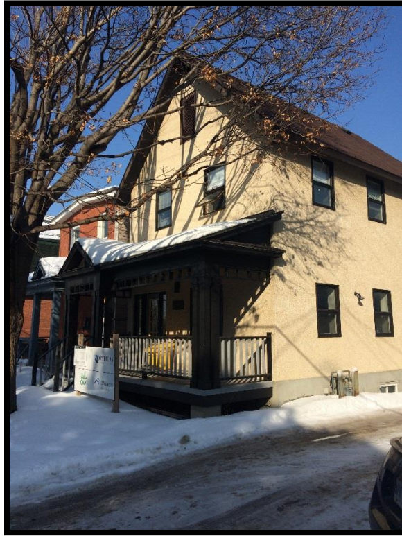
Photograph 1: View of the west building face.
