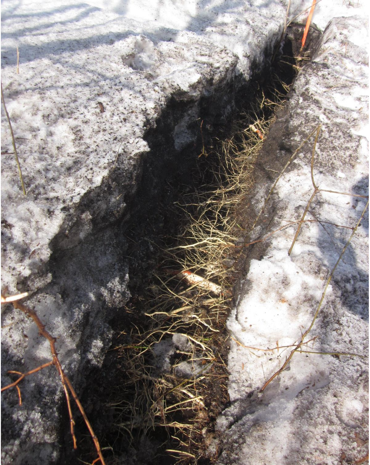
Picture 1. Results of hydro excavation 7.8m from tree #38 (photo taken March 2020).
