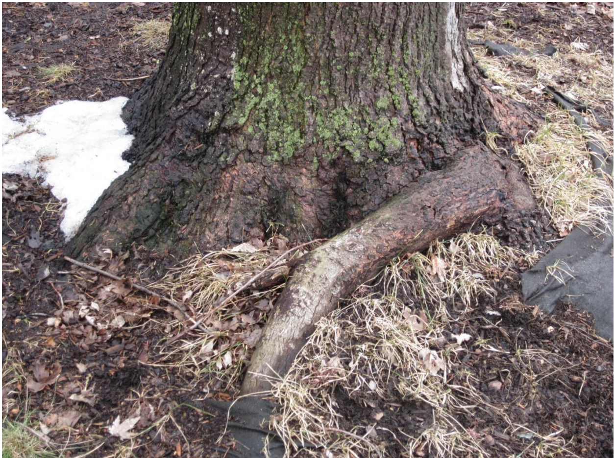
Picture 1. Binding root on root collar of tree in Phase 2 of Qwest development. Picture taken March 2018.
