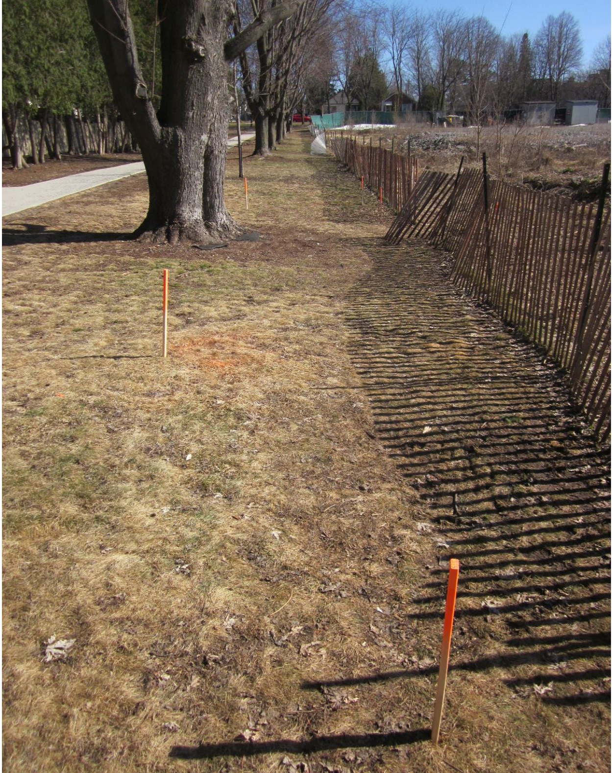
Picture 3. Line of silver maple trees in Phase 2 of Qwest development (looking southeastward). Snow fence is approximate distance of excavation in relation to trees in background (tree #41 is in foreground). Picture taken April 2019.
