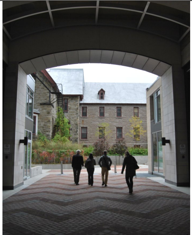
Photo 2: View of Monastery through west arch of Phase I of development.
