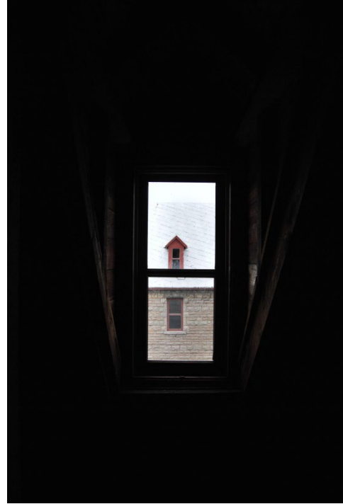
Photo 23: View out of typical dormer facing towards courtyard (dormers to be removed and replaced with contemporary dormers in proposed development).
