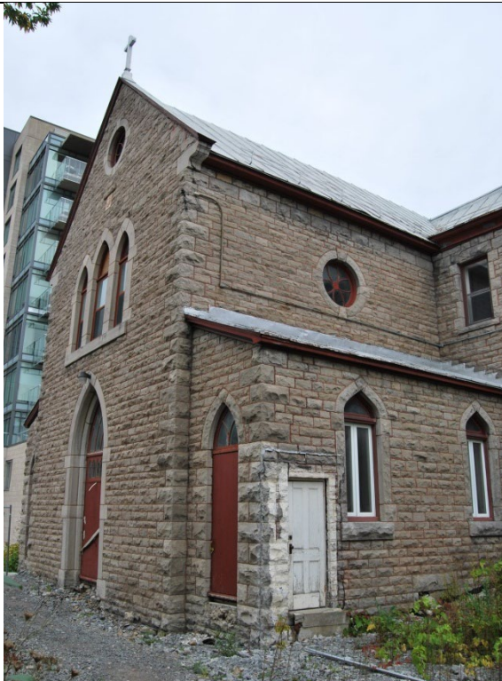
Photo 7: View of the Chapel from the southwest (to be rehabilitated in proposed development).
