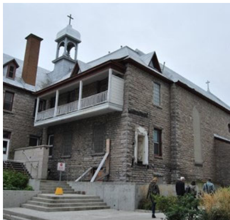
Figure 8: Bellcote at rear of chapel.
