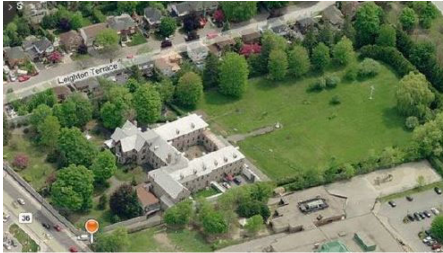
Figure 2: View of the site prior to development.
