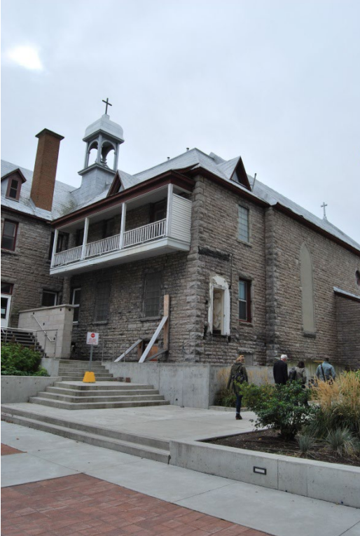
Photo 5: View of the southern wall of Chapel with gallery (area to be rehabilitated as part of proposed development).
