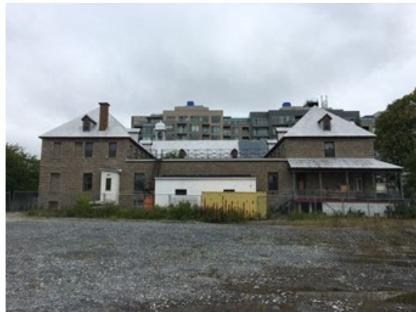
Figure 9: South face of monastery.
