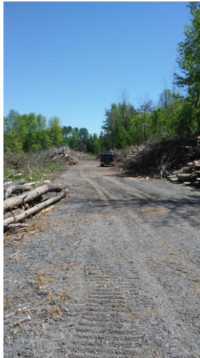
Photo 2: On-site construction laneway, view from Franktown Road
