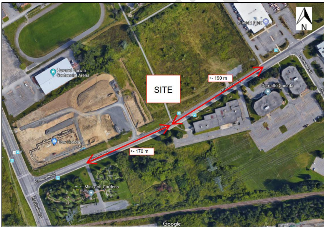
Figure 3.5: Adjacent Driveways (Courtesy of Google Earth)
