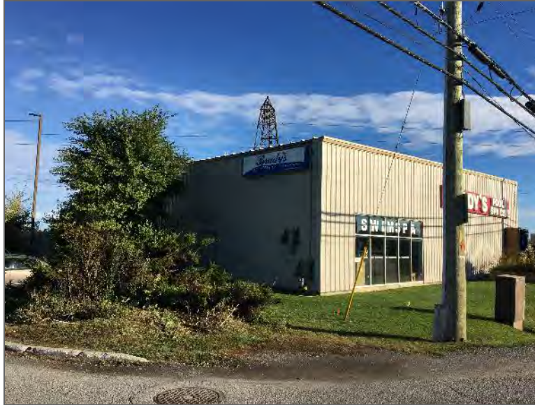
Photo 3 – Looking northeast from the south elevation of the Phase One Property.
