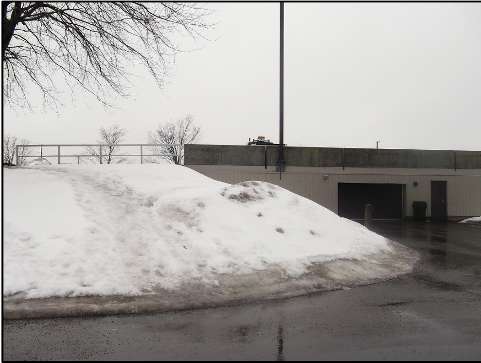
Photograph 4: View of the eastern face of the adjacent parking structure, facing northwest.
