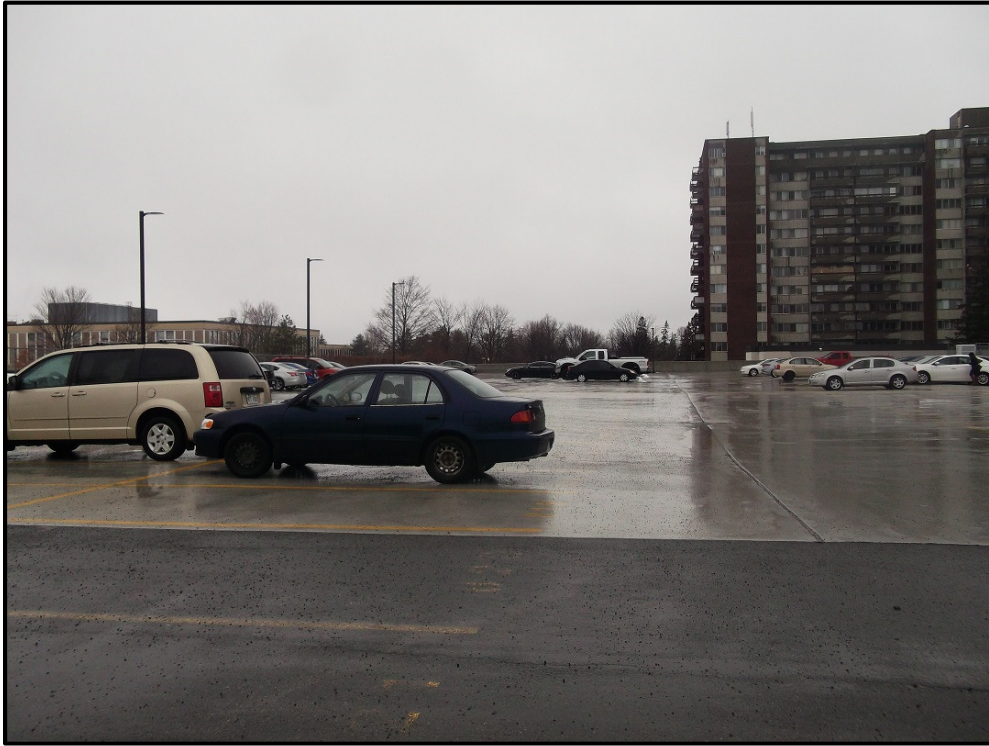
Photograph 3: View of the adjacent parking garage structure to the north, facing north.
