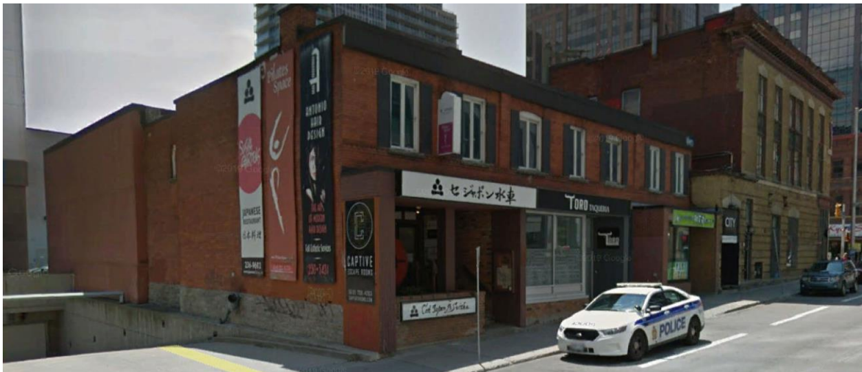
Figure 9: View looking east on Slater to the development site. Note the projecting brick walls enclosing the storefronts. Note the east wall (left) and the stone foundation walls that delimit the original built plan. The rear addition evident to the left of the photograph was completed circa 1956. Source: Google Earth
