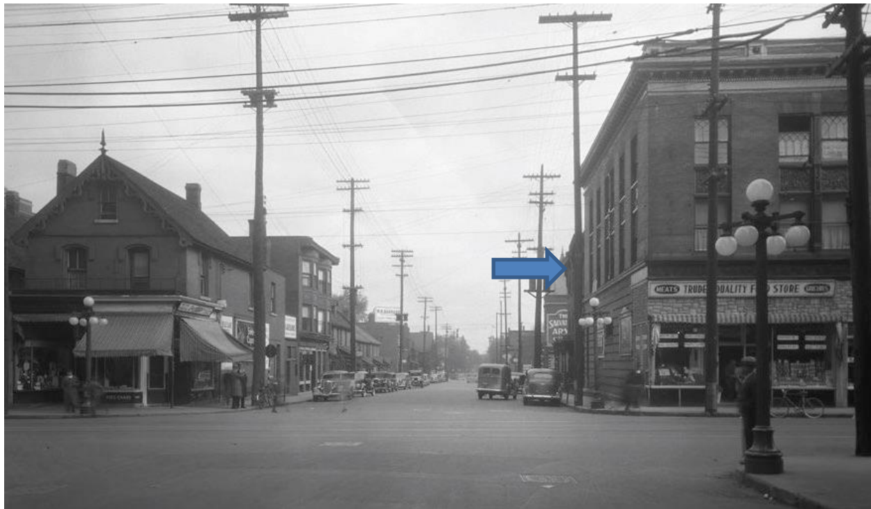
Figure 14: 1938 view looking east on Slater from Bank Street. The building on the development site is arrowed. The building is clearly three storeys in height, and has a strong cornice overhang. One storey entrance bays enclosed with roof structures extend to the property line. Source: Library and Archives Canada Mikan No. 4169733
