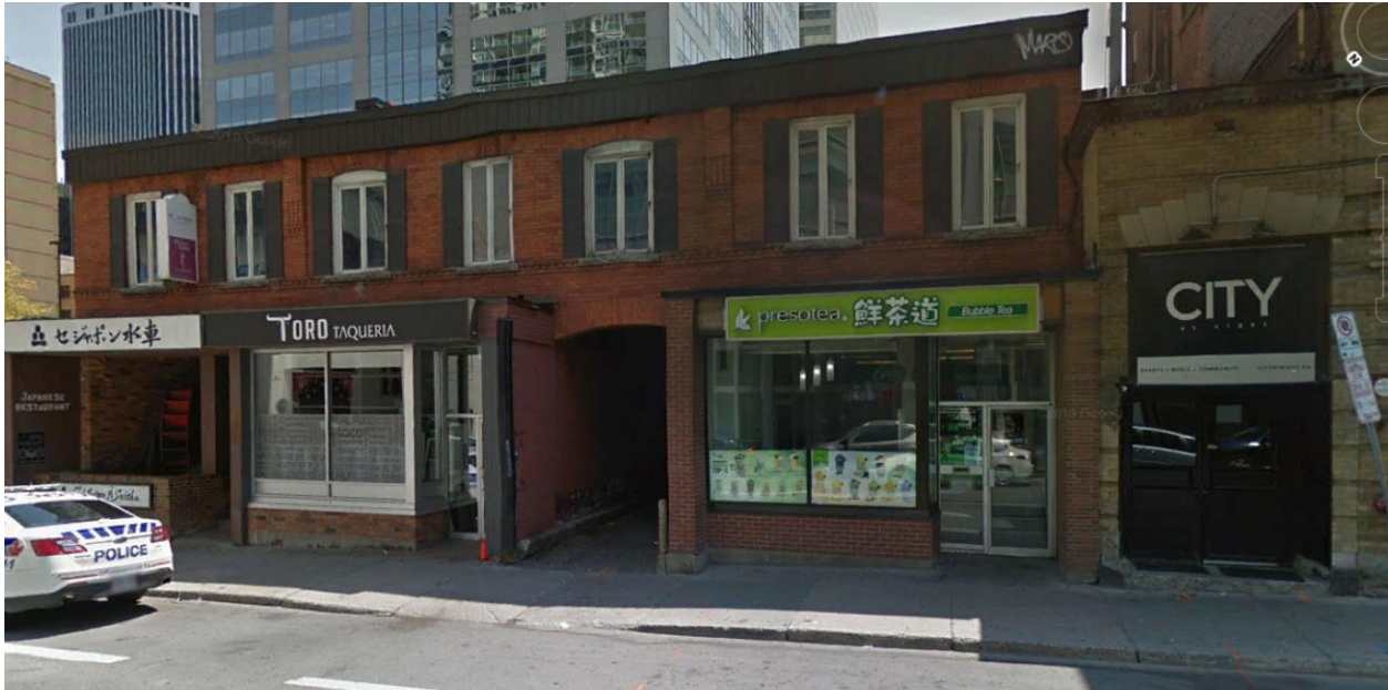
Figure 7: View of 208 – 212 Slater. Note the carriageway and the projecting brick walls enclosing the ground floor commercial storefronts presumably installed in 1968 (HSF). The property is categorized as a Group 3 heritage resource. Note the single storey wing at the rear of 129 Bank St. Source: Google Earth
