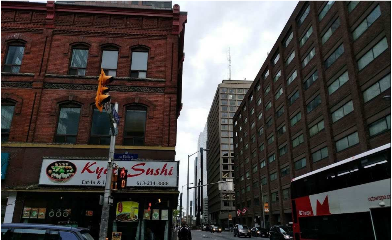
Figure 7: View to the west of the subject property
