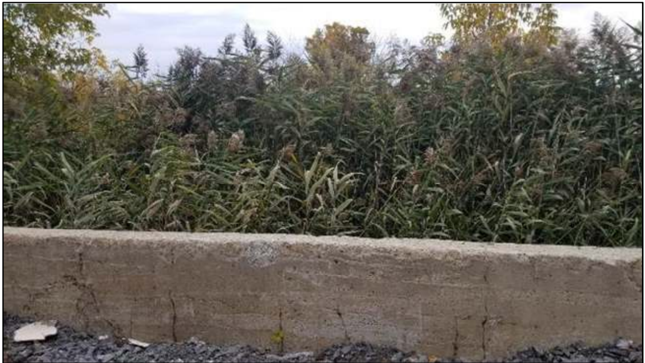
Figure 4: Retaining Wall at North East Side of Property
