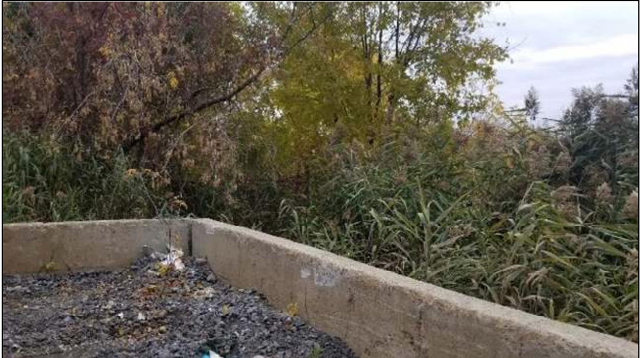
Figure 3: Retaining Wall at North East Side of Property
