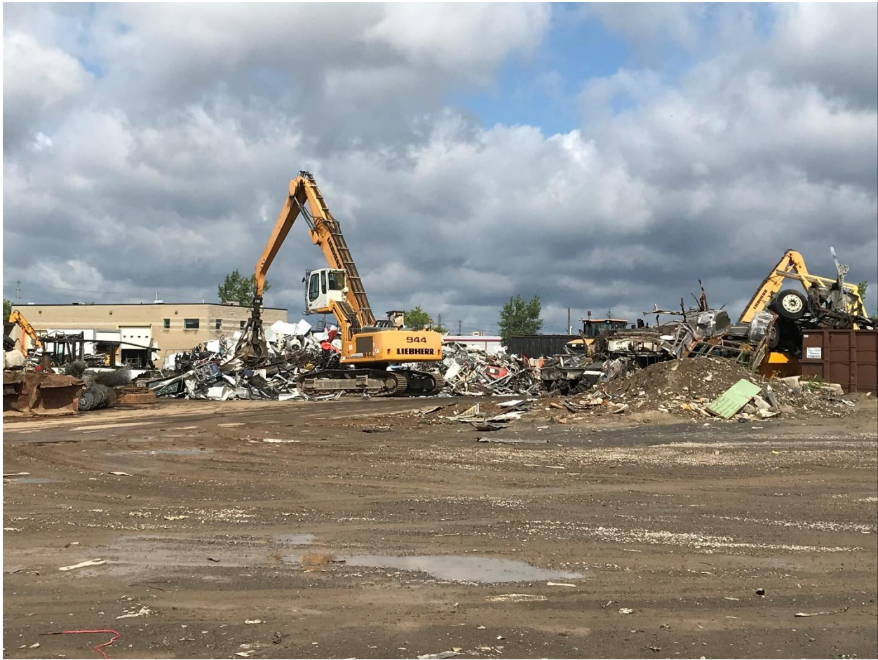
Photograph 16: Looking northwest over the Site from the southeast corner (August 2019).
