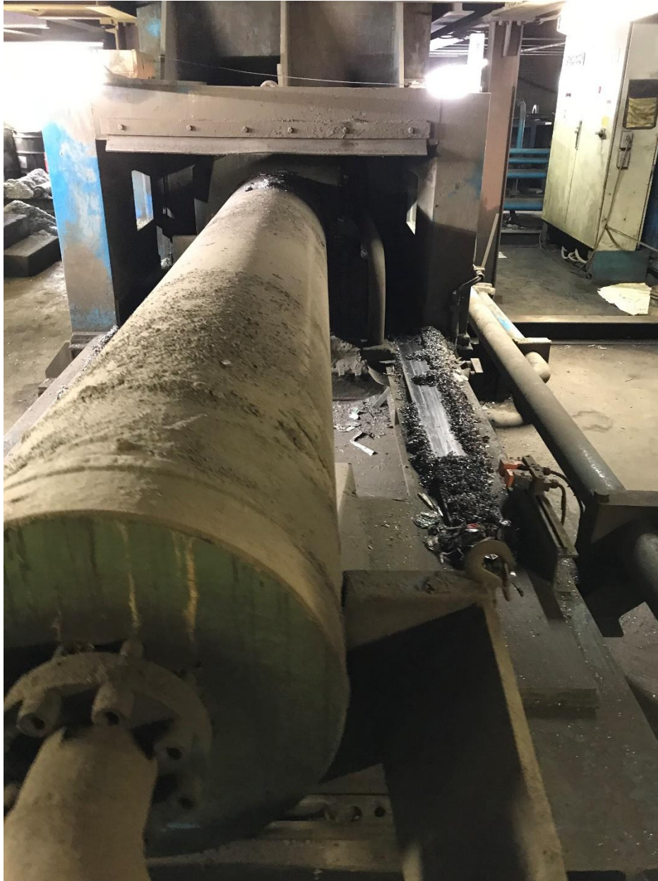
Photograph 7: Looking west along the hydraulic piston of the hydraulic bailer located in the southwest corner of the Main Building (August 2019).
