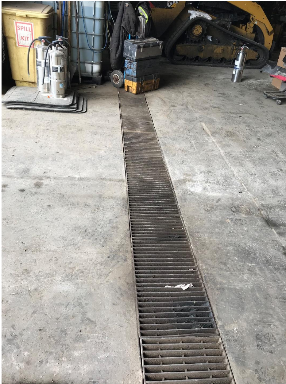
Photograph 24: Looking west at the linear drain on the south side of the Garage Building. The drain discharges to a holding tank that is emptied on an as needed basis (August 2019).
