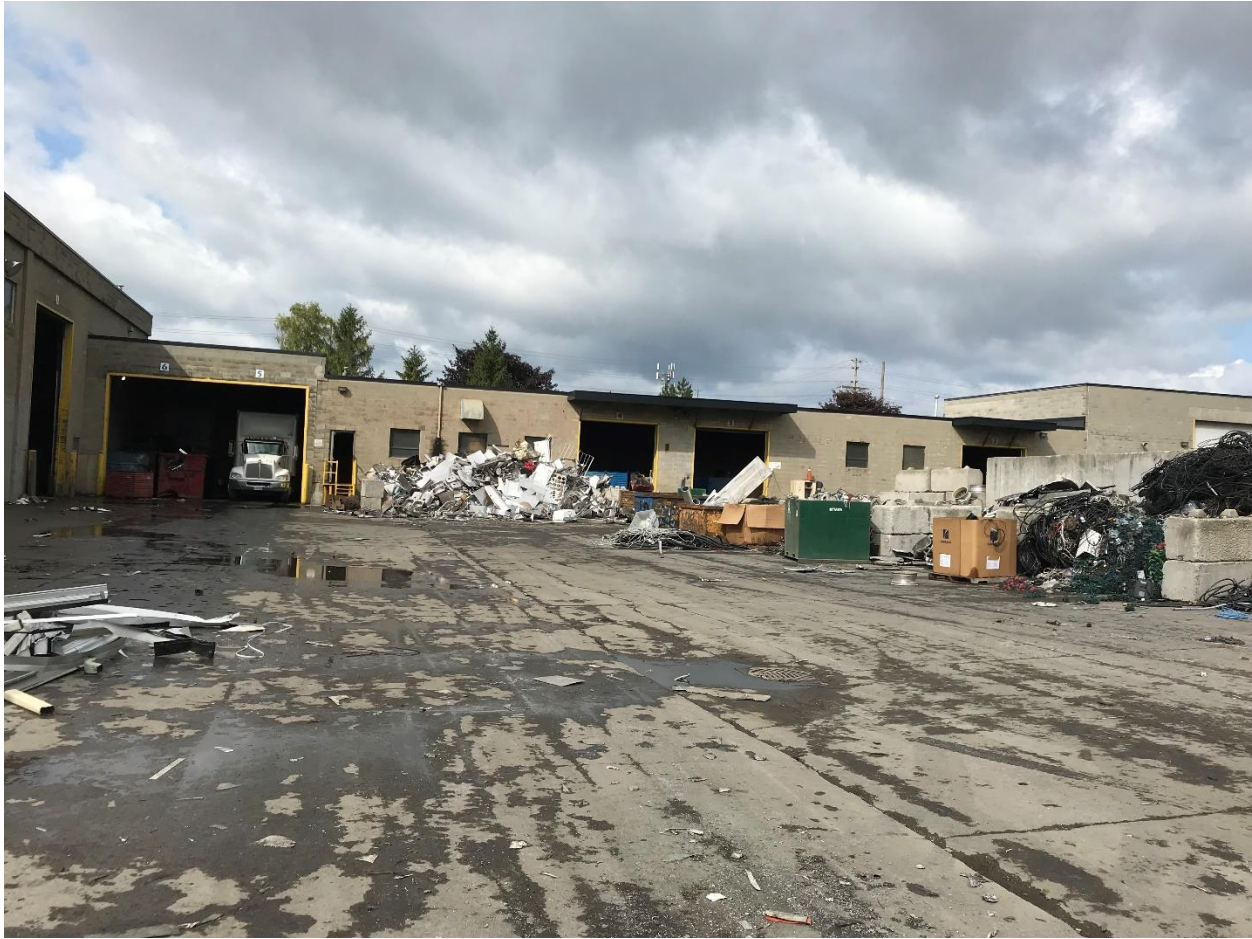
Photograph 9: Looking west at the east elevation of the north branch of the Main Building. The center portion is the original building constructed prior to 1965 (August 2019).
