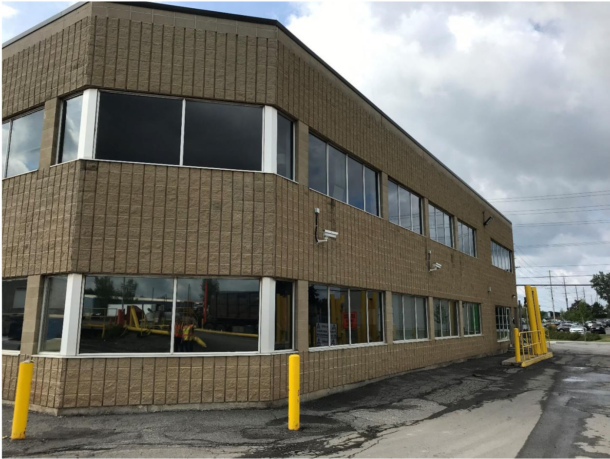
Photograph 26: Looking southwest at the northern end of the Main Building, at the offices built in 1998 (August 2019).
