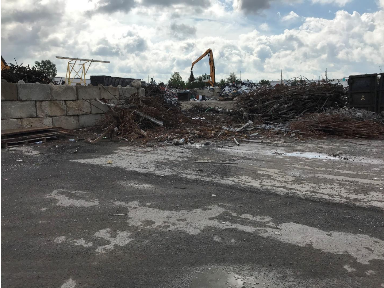
Photograph 19: Looking southeast across the Site from the northwest corner (August 2019).
