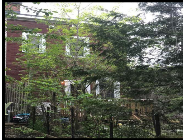
Photo 2: The Phase One Property (24 Pretoria Avenue – south facing exterior wall)
