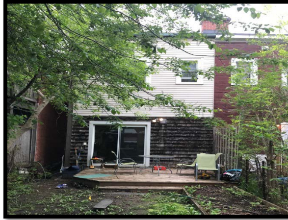
Photo 8: The Phase One Property (26 Pretoria Avenue – south facing exterior wall)
