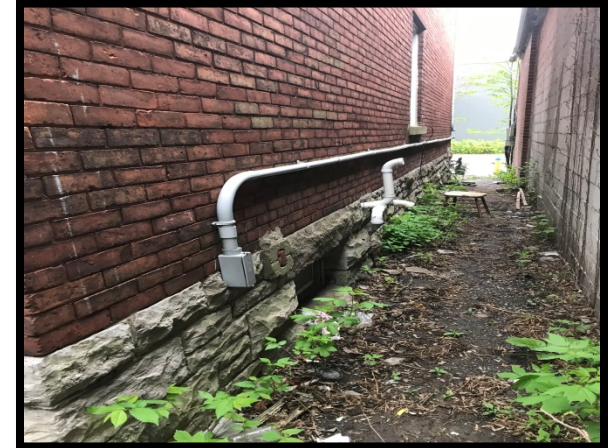
Photo 3: The Phase One Property (24 Pretoria Avenue – east facing exterior wall)
