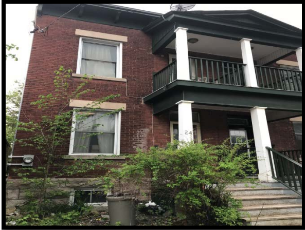
Photo 1: The Phase One Property (24 Pretoria Avenue – north facing exterior wall)
