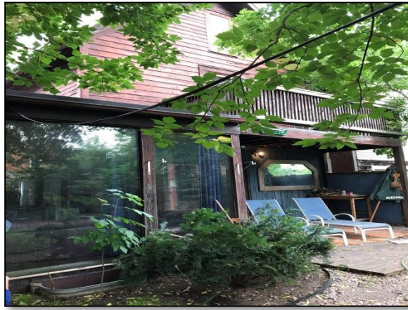
Photo 2: The Phase One Property (28 Pretoria Avenue – south facing exterior wall)
