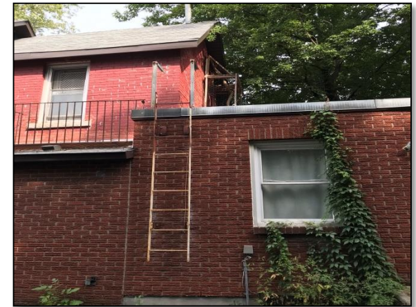
Photo 12: The Phase One Property (30 Pretoria Avenue – west facing exterior wall)
