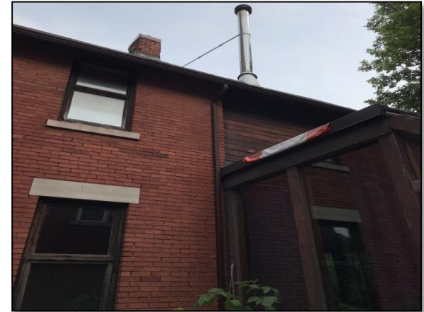
Photo 3: The Phase One Property (28 Pretoria Avenue - west facing exterior wall)
