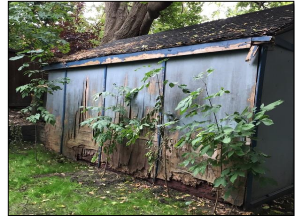
Photo 6: The Phase One Property (28 Pretoria Avenue – detached garage)
