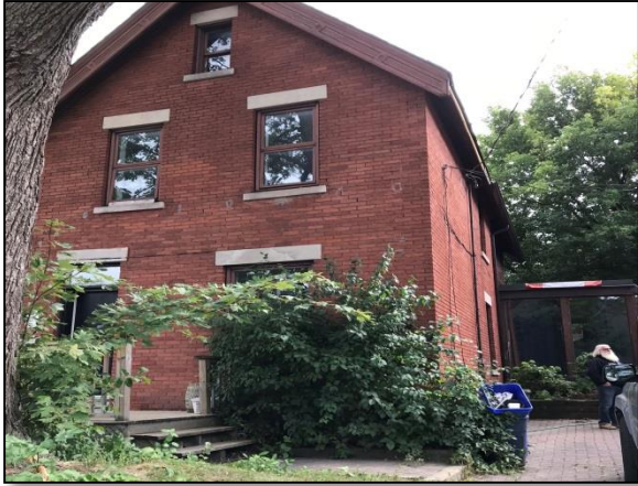
Photo 1: The Phase One Property (28 Pretoria Avenue – north facing exterior wall)
