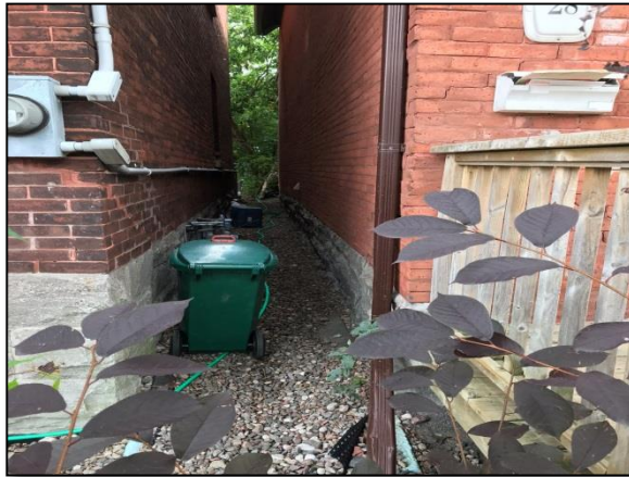
Photo 4: The Phase One Property (28 Pretoria Avenue – east facing exterior wall)
