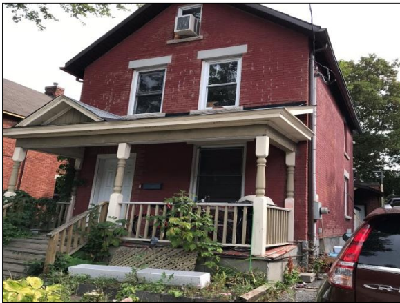
Photo 10: The Phase One Property (30 Pretoria Avenue – north facing exterior wall)
