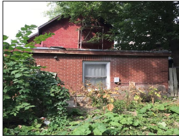
Photo 11: The Phase One Property (30 Pretoria Avenue – south facing exterior wall)
