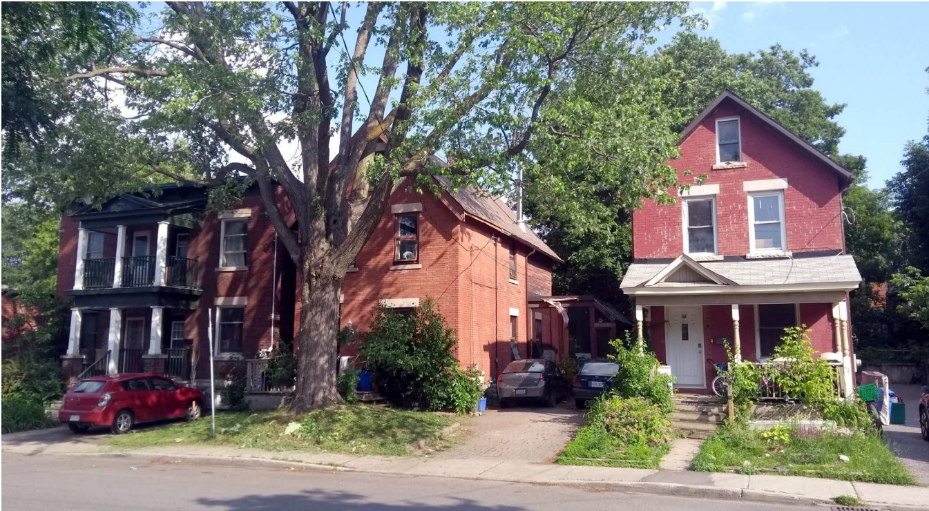
Figure 5: Site Photo, Fotenn Consultants 2019-07-02
