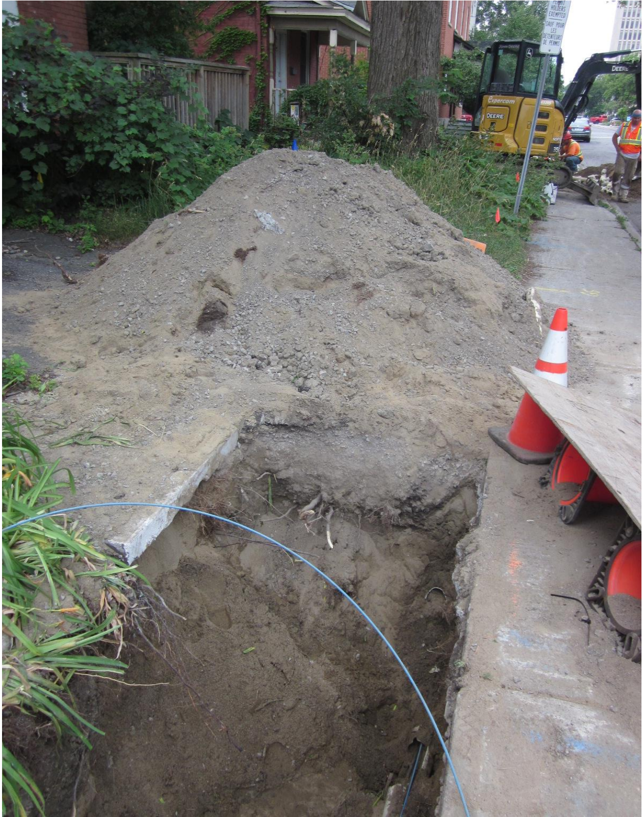
Picture 2. Recent root damage within maple's critical rooting zone due to work on Bell lines (taken July 2020)
