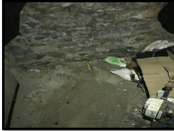
Photo 2: The Phase One Property (24 Pretoria Avenue – basement floor near furnace)
