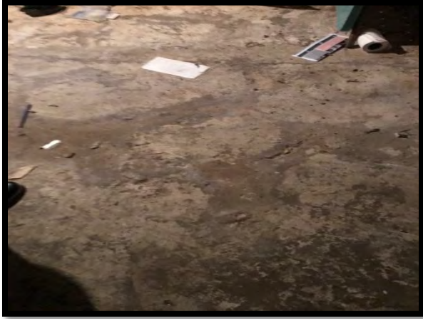
Photo 1: The Phase One Property (24 Pretoria Avenue – basement floor near furnace)
