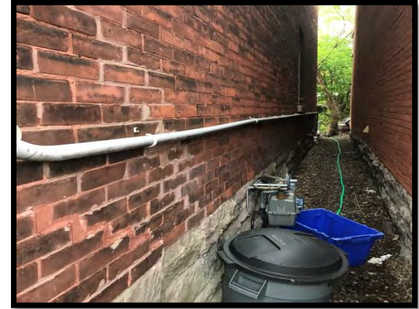
Photo 9: The Phase One Property (26 Pretoria Avenue – west facing exterior wall)
