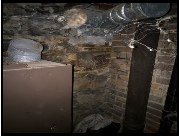
Photo 4: The Phase One Property (24 Pretoria Avenue – basement wall behind furnace)
