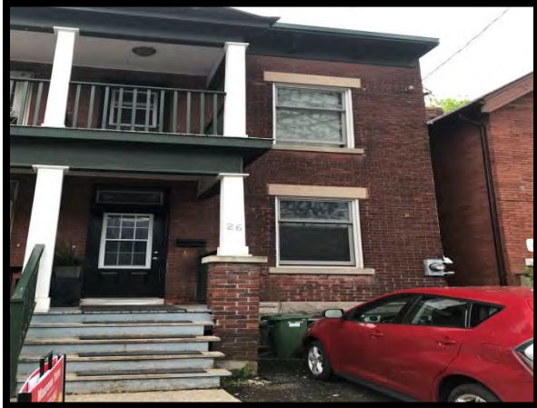
Photo 7: The Phase One Property (26 Pretoria Avenue – north facing exterior wall)
