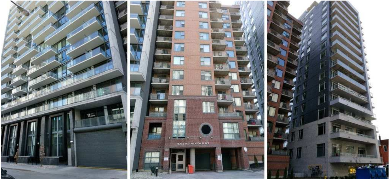
Figure 4: View to the south of the subject property
