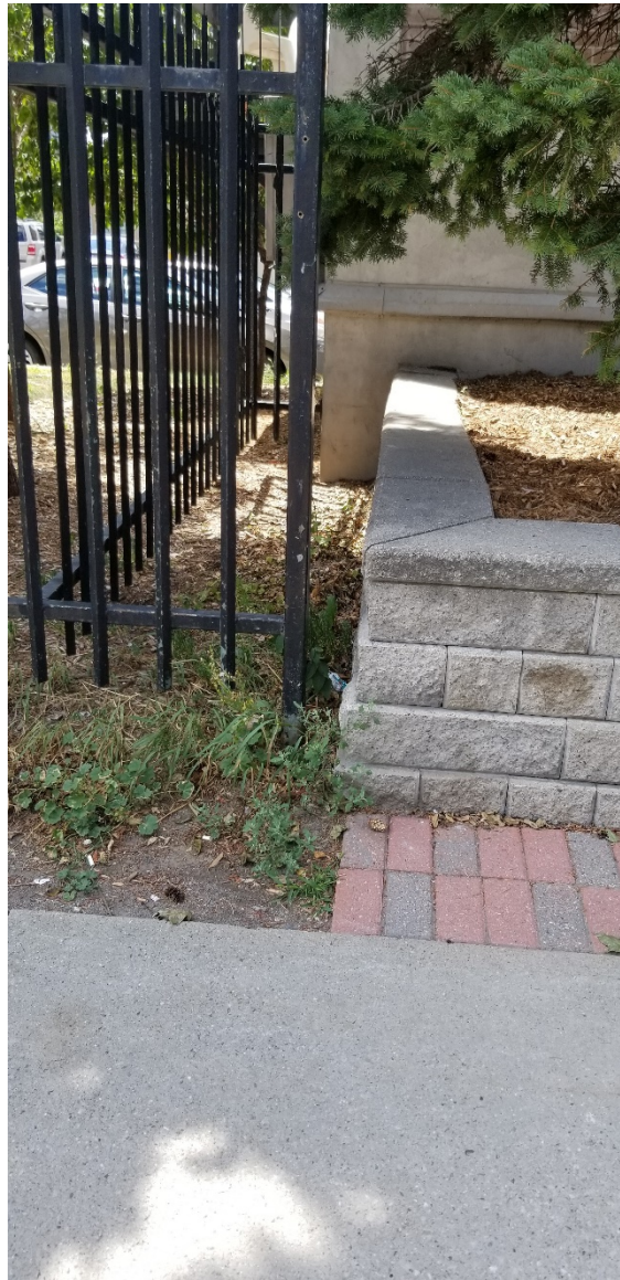
Corner of 360 Bell retaining wall
