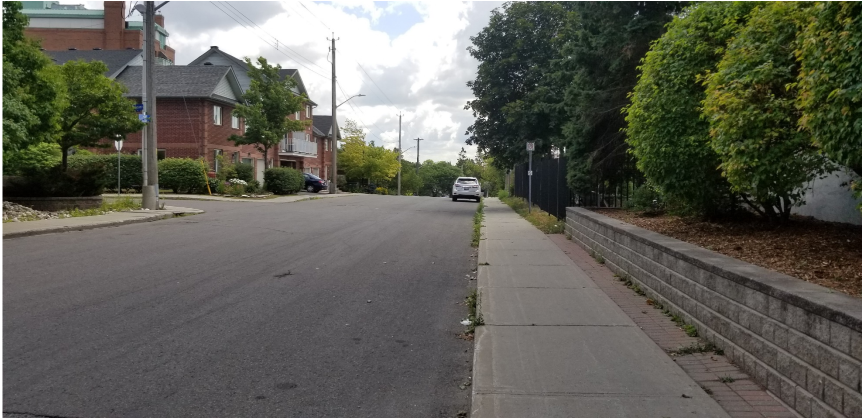
Photo from manhole / fire hydrant on opposite side of Bell St, looking south on Bell St.
