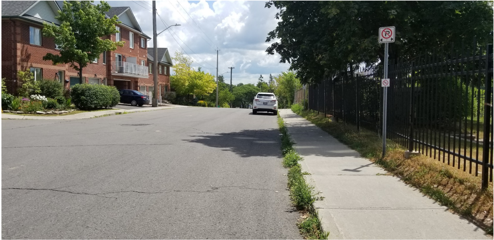
Photo from corner of retaining wall, looking south on Bell St.
