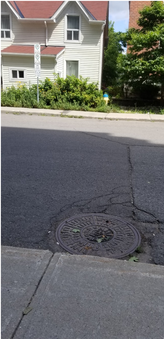
Manhole/Hydrant in front of UPS truck
